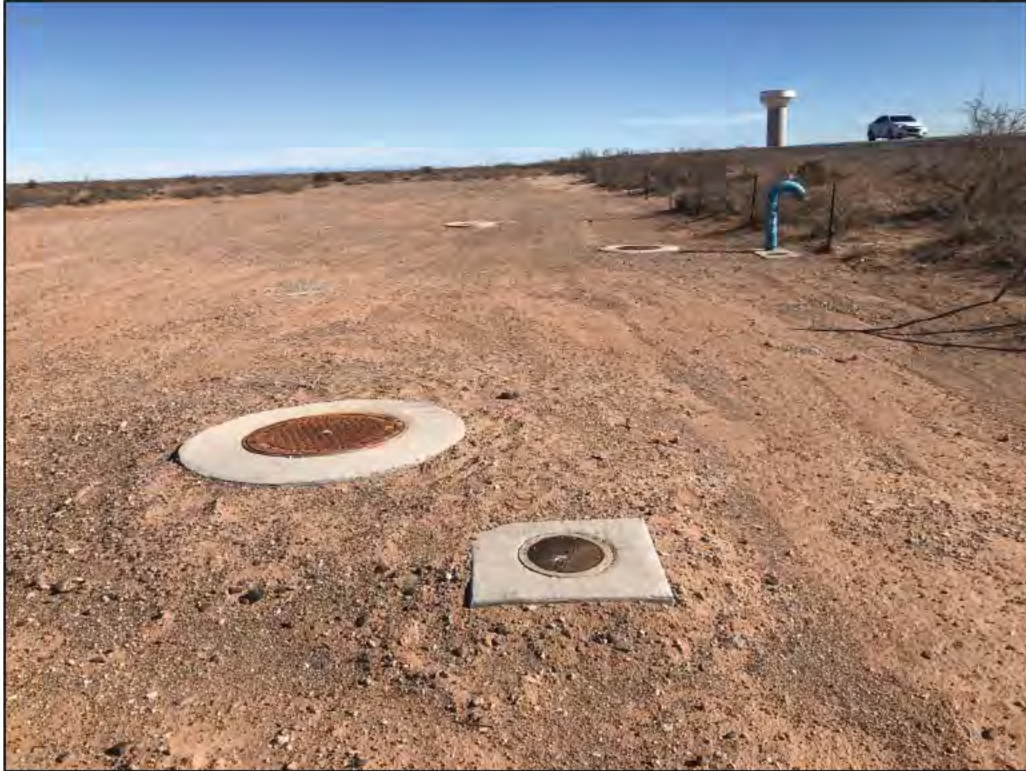
Photograph 3. Underground utilities installation located along the southern boundary of the proposed project area.
