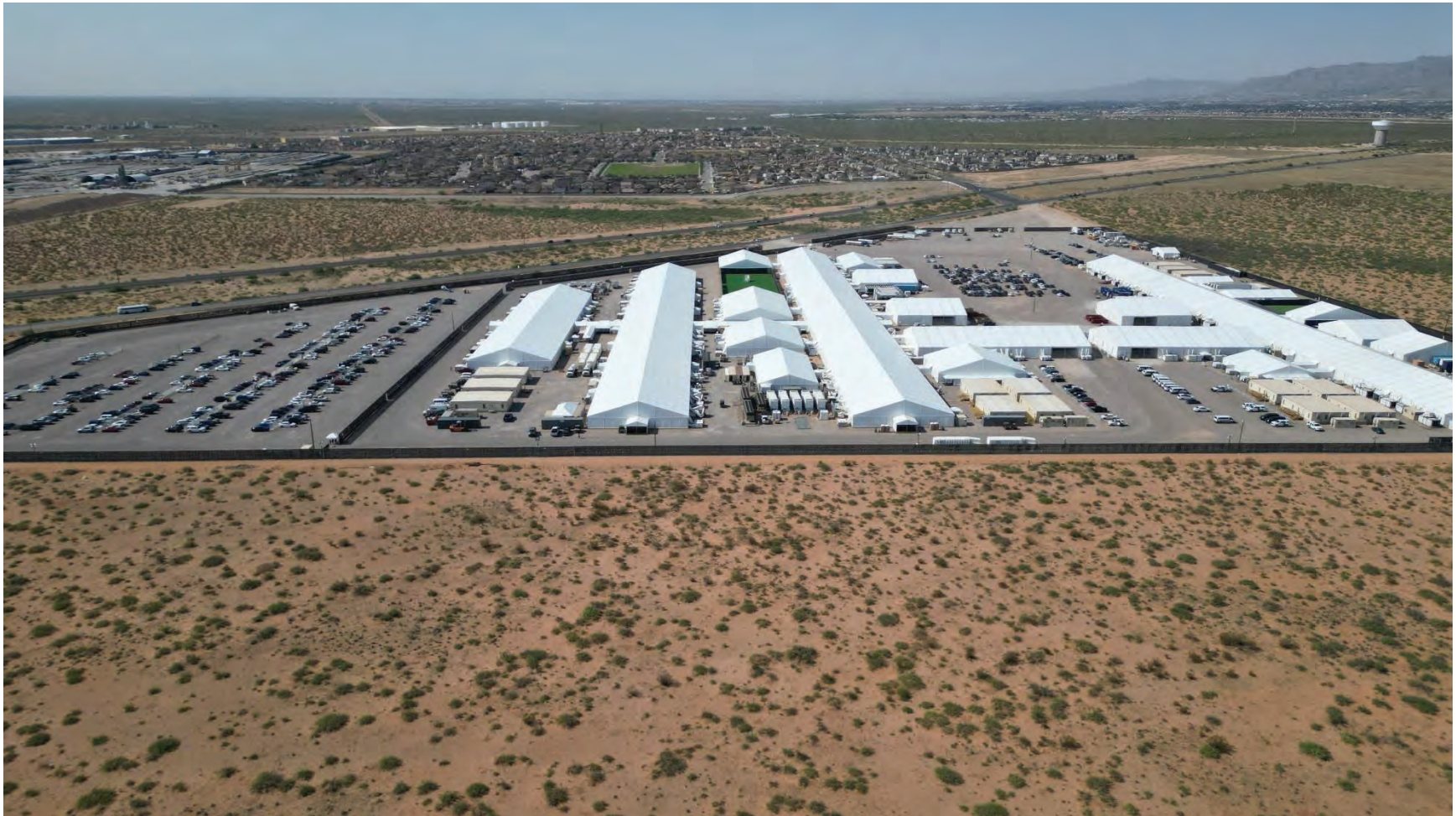
Figure 3: Existing Project Site Location, Facing East
