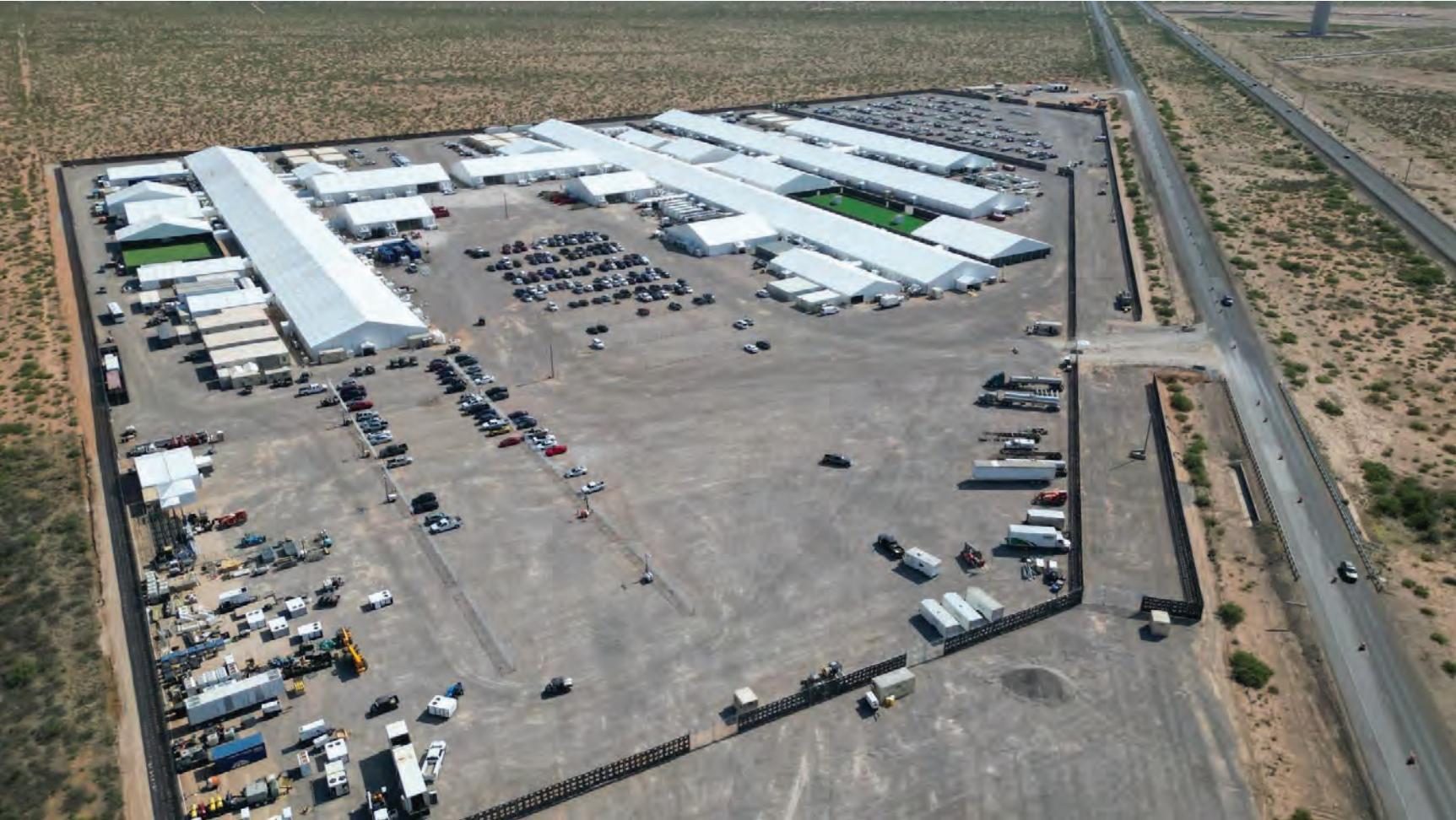
Figure 2: Existing Project Site Location, Facing North
