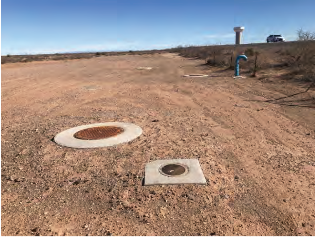
Underground utilities located along southern property boundary, adjacent to Highway 54.
