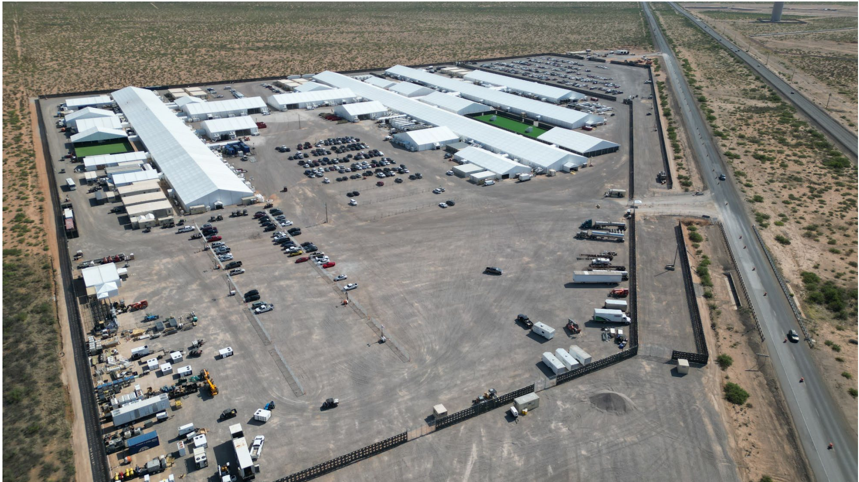
Figure 1-2: View of Project Site, Facing Northeast
