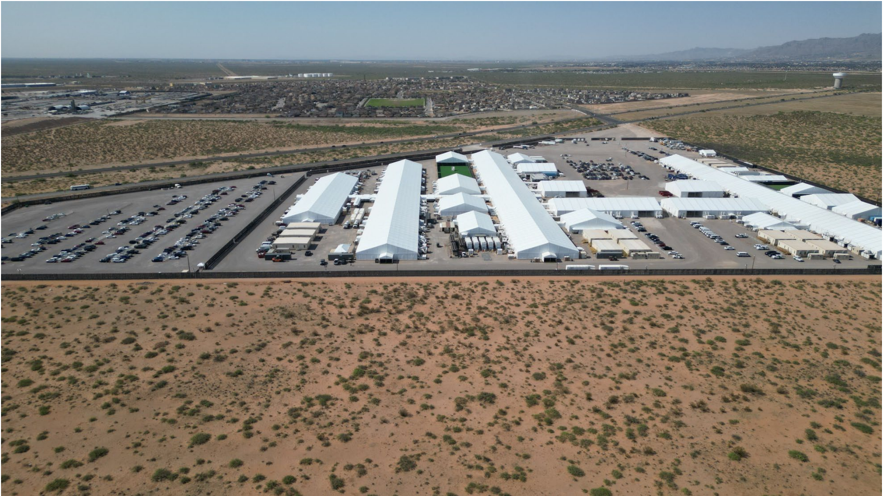
Figure 1-3: View of Project Site, Facing South
