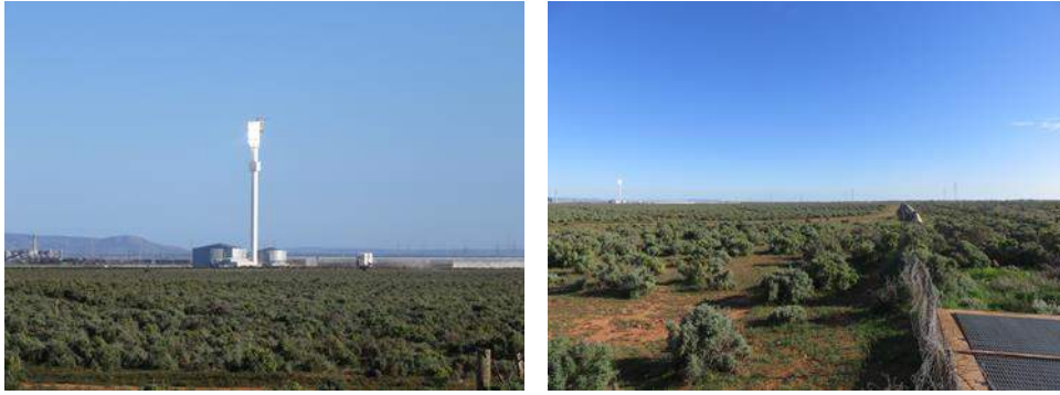
Figure 7 Sundrop Farm Solar Array Tower
