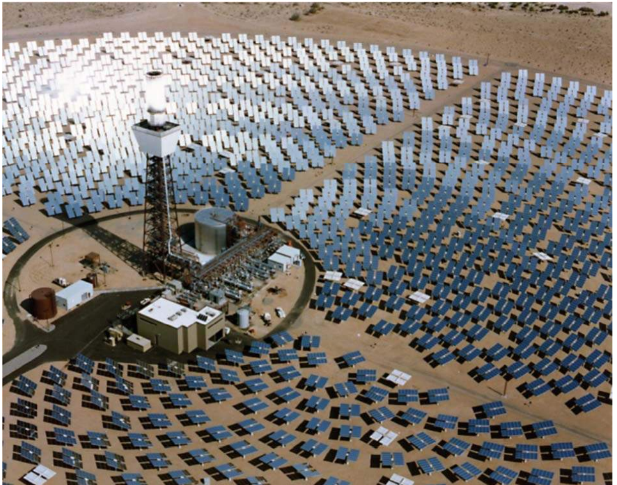
Figure 8-2 An example of glare from the receiver and heliostat field (SolarReserve)
