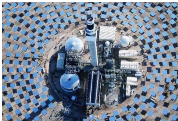
Figure 3-6 Crescent Dunes Solar Energy Project, Nevada – Tower, plant and Heliostats
