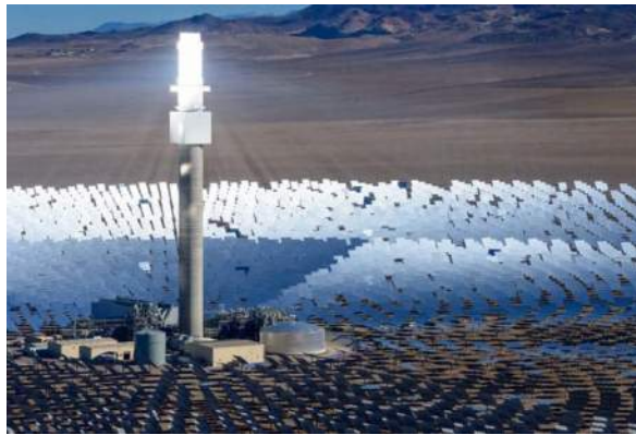
Figure 3-4 Crescent Dunes Solar Energy Project, Nevada - Molten salt receiver tower
