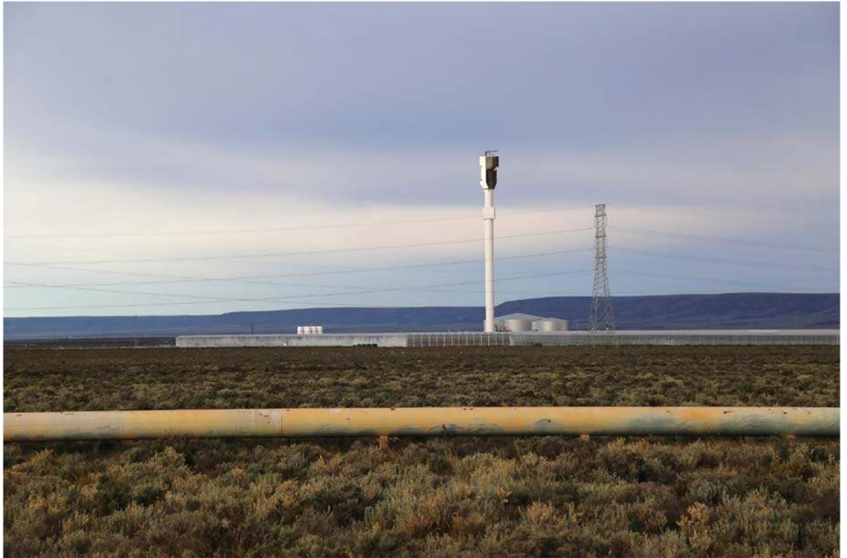
Figure 8-3 Sundrop Farms Renewable Energy facility
