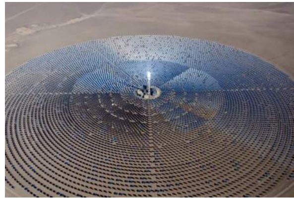
Figure 3-5 Crescent Dunes Solar Energy Project, Nevada – Heliostat array
