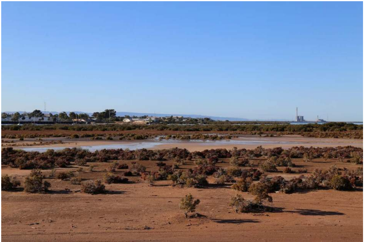
Figure 4-2 Northern Power Station seen from 7 km away (moderately prominent)
