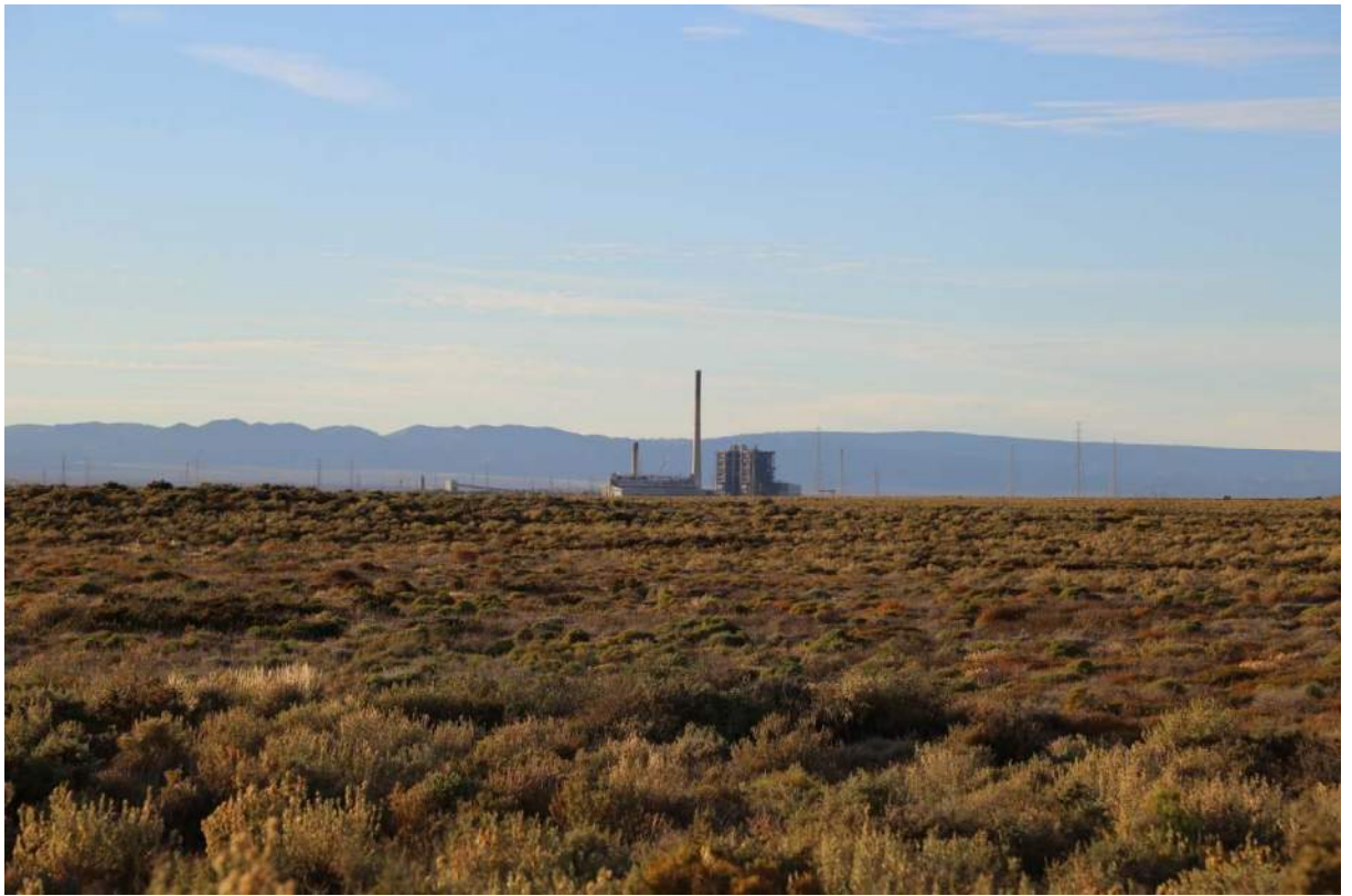
Figure 4-1 Northern Power Station seen from 4 km away (visually prominent)
