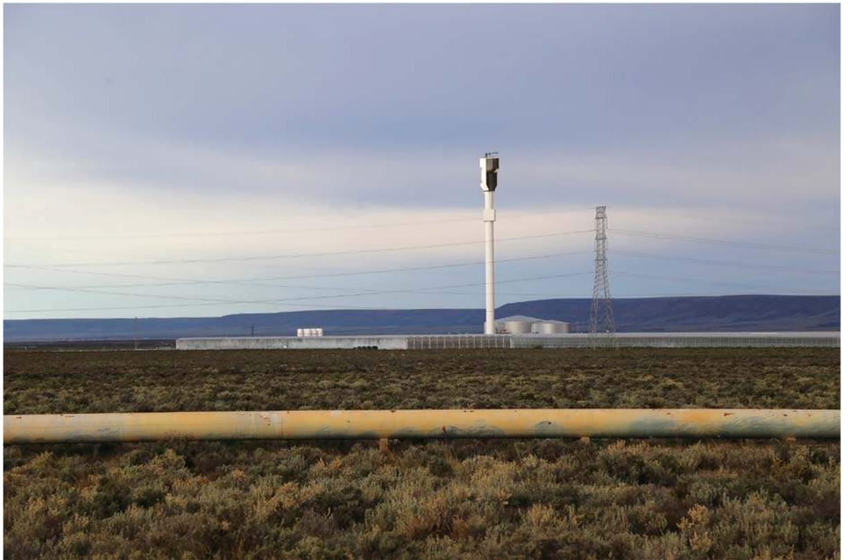
Figure 6-16 Sundrop Farms Renewable Energy facility from Princes Highway
