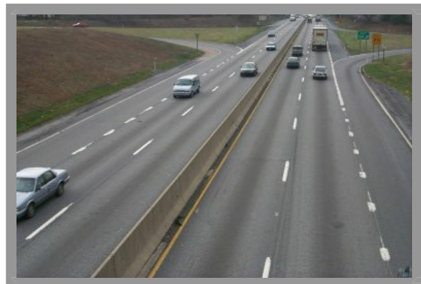
Figure 6-8 Type 2: Fixed Barrier
