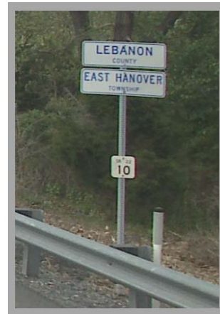
Figure 10-6 Boundary with Segment Sign
