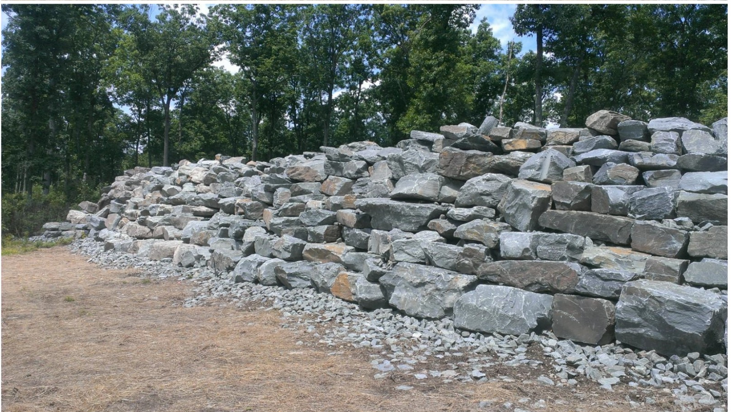
Here is another example of an eastern small-footed bat roost structure. This structure was constructed away from the tree line to ensure adequate solar exposure.
