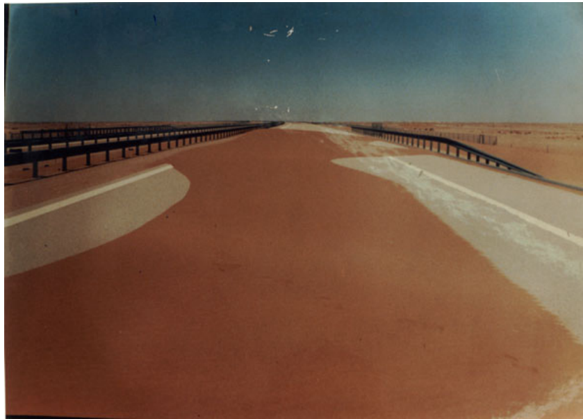
Figure 2: Creeping sands cover the highways creating a serious hazard
