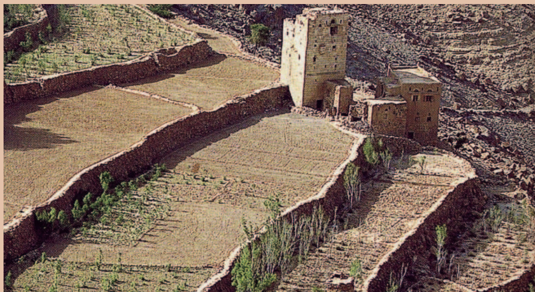
Yemen, terracing system for the protection and cultivation of the slope. The water intakes deviate the flows from their natural course and direct them along the walls on the terraces. Towers and stone buildings are placed to defend the cultivations. Photo: P. Laureano.
