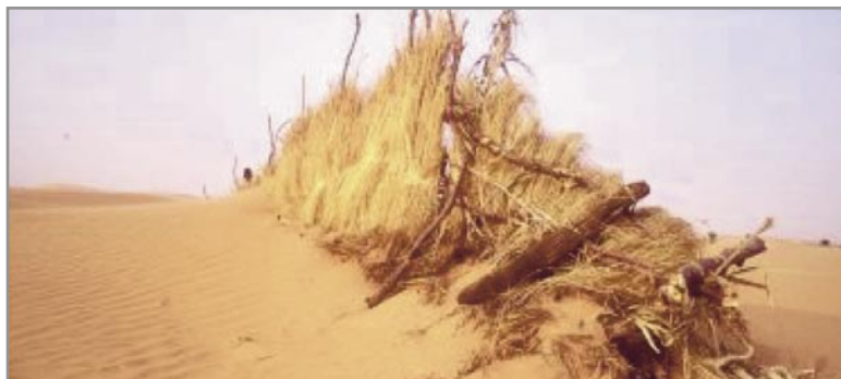
Zer-El-Ghilbi oasis, Mauritania. In an attempt to block the shifting sand, barriers are made from palm leaves. Photo: I. Balderi. FAO/18833.
