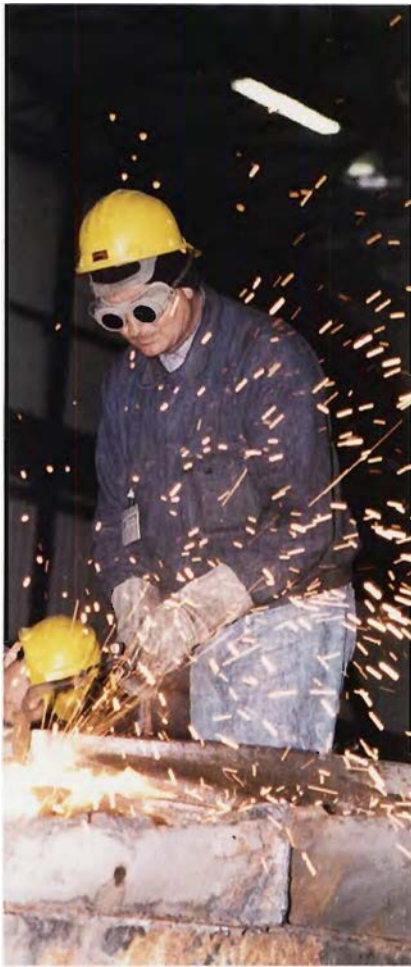
Severing was the primary reduction method for all treaty-limited equipment (TLE).
