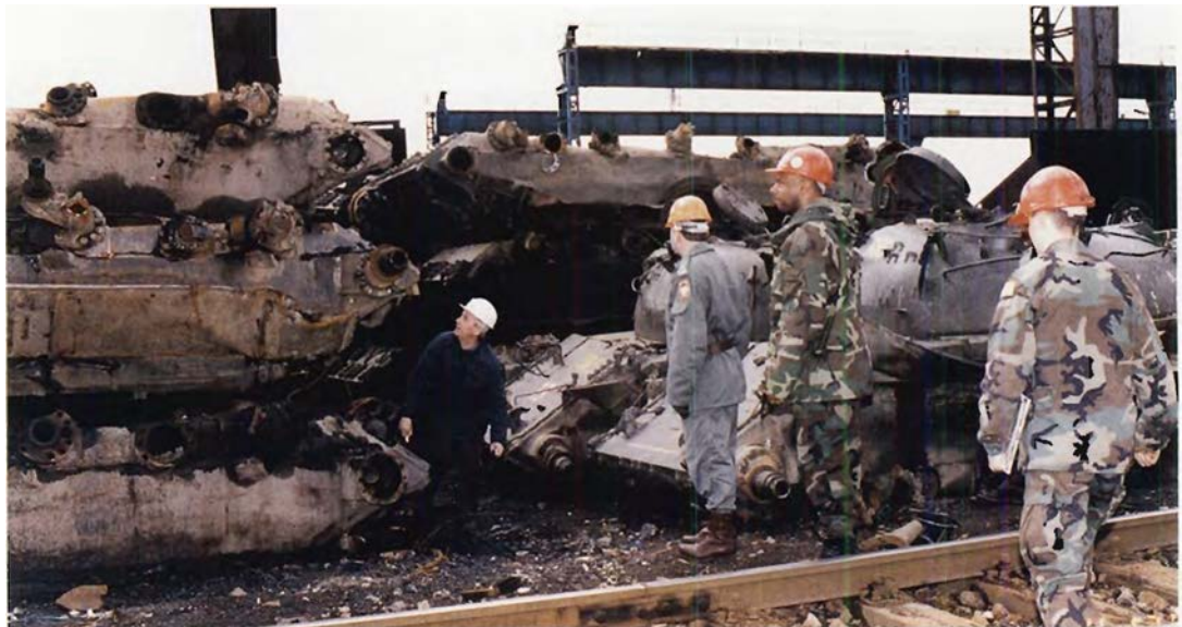
Poland's eight-ton ball crushed TLE efficiently and economically.
