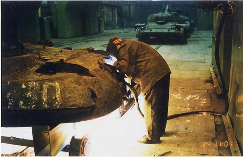
Severing of a turret in Belarus.
