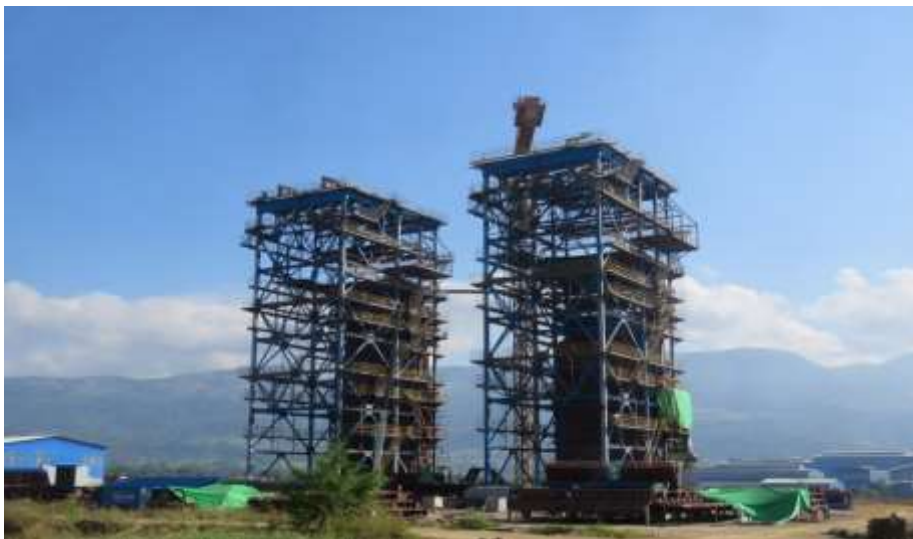
Figure – 21: Boilers in the process of construction
