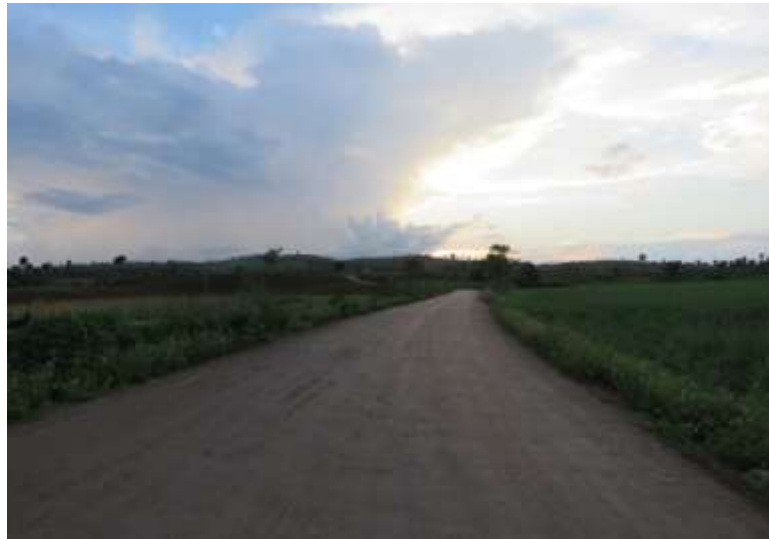
Figure – 92: Bantbwe-konkyi-taungkya-innwine road constructed by the company
