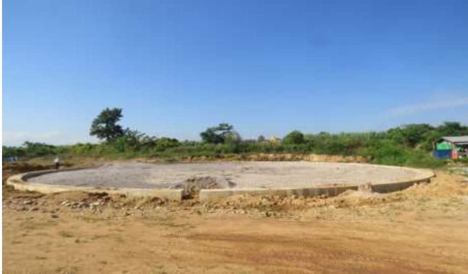
Figure – 19: Molasses tank area in the process of construction
