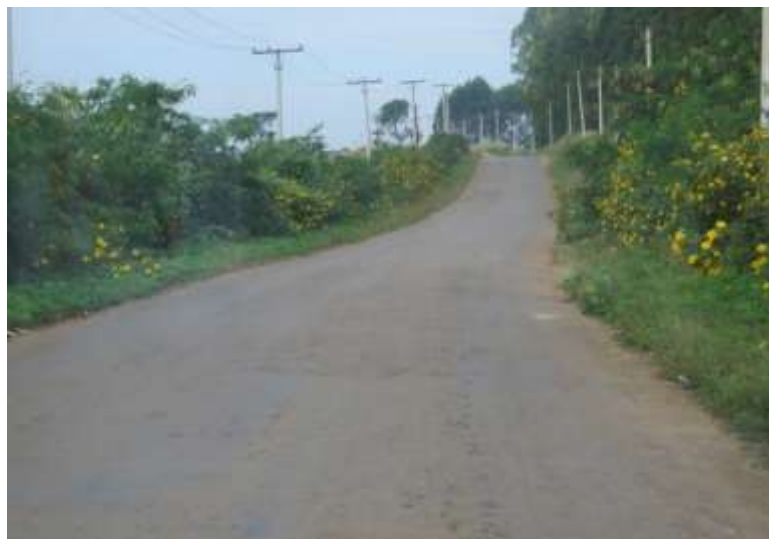
Figure – 93: Le-gynn-gwae road constructed by the company
