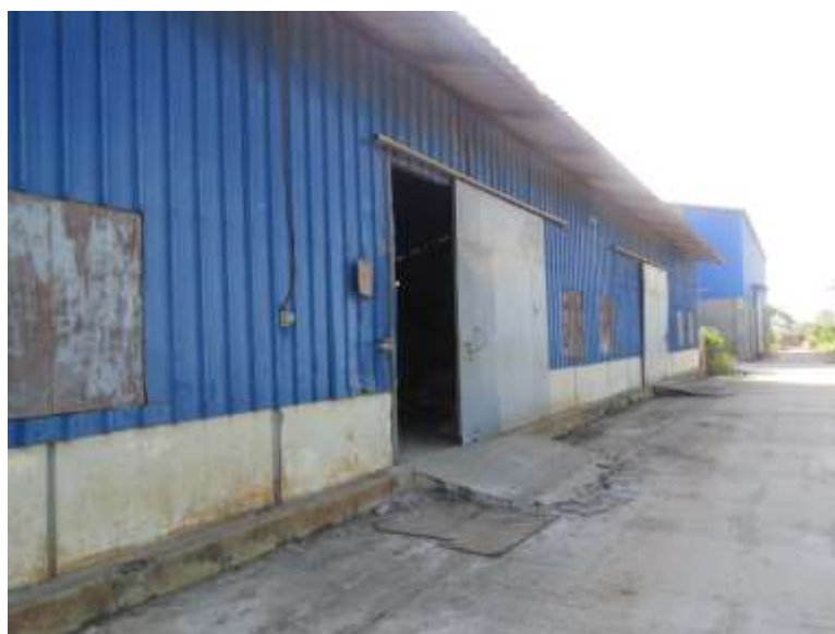
Figure – 30: Chemical store inside factory 2 premise
