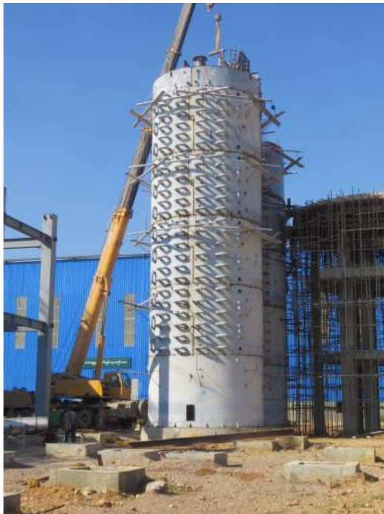
Figure – 18: Vertical crystallizer in the process of construction
