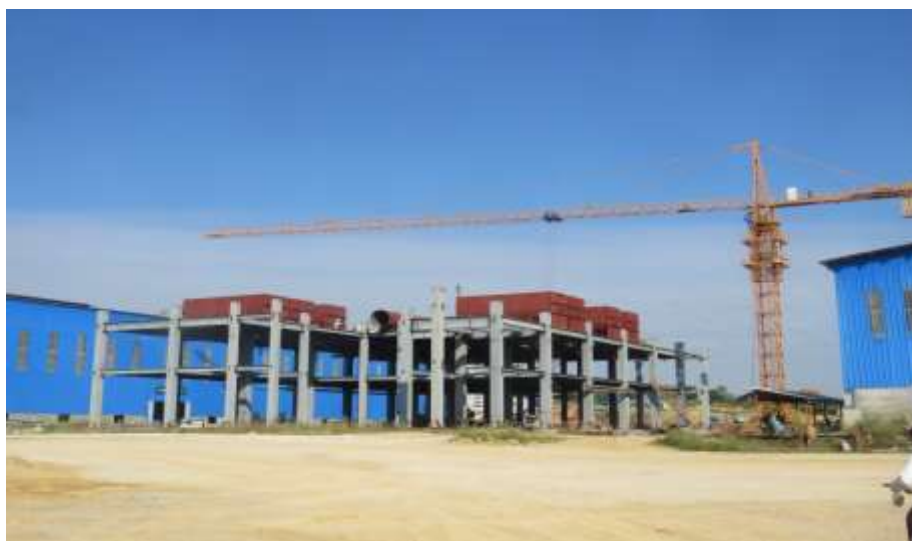
Figure – 13: Process house in the process of construction
