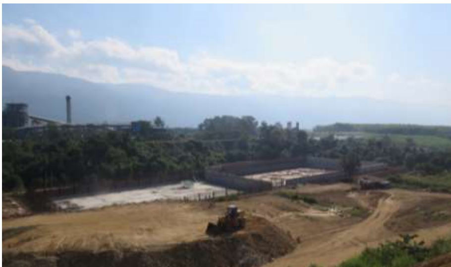
Figure – 24: Cooling tower area in the process of construction
