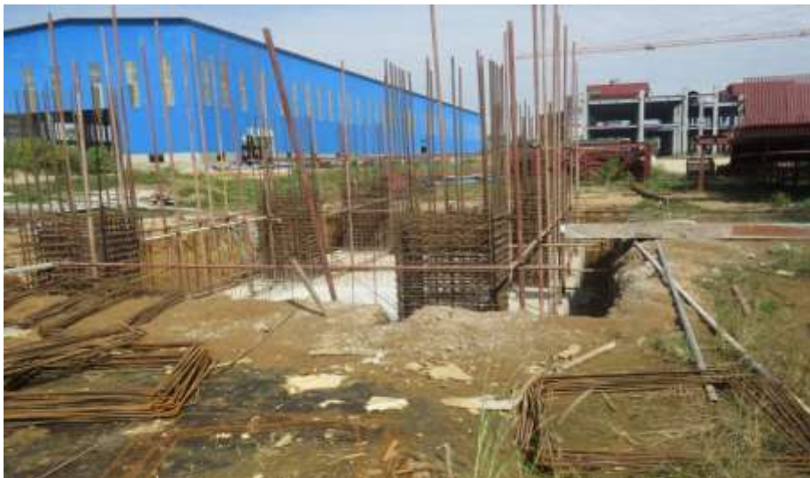
Figure – 20: Turbine house area in the process of construction
