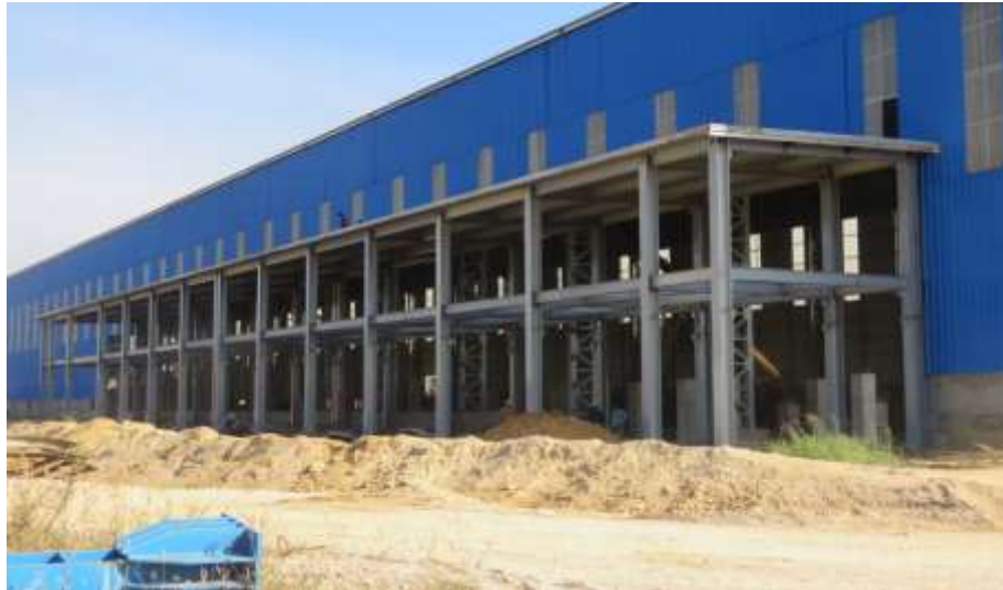
Figure – 14: Control room in the process of construction
