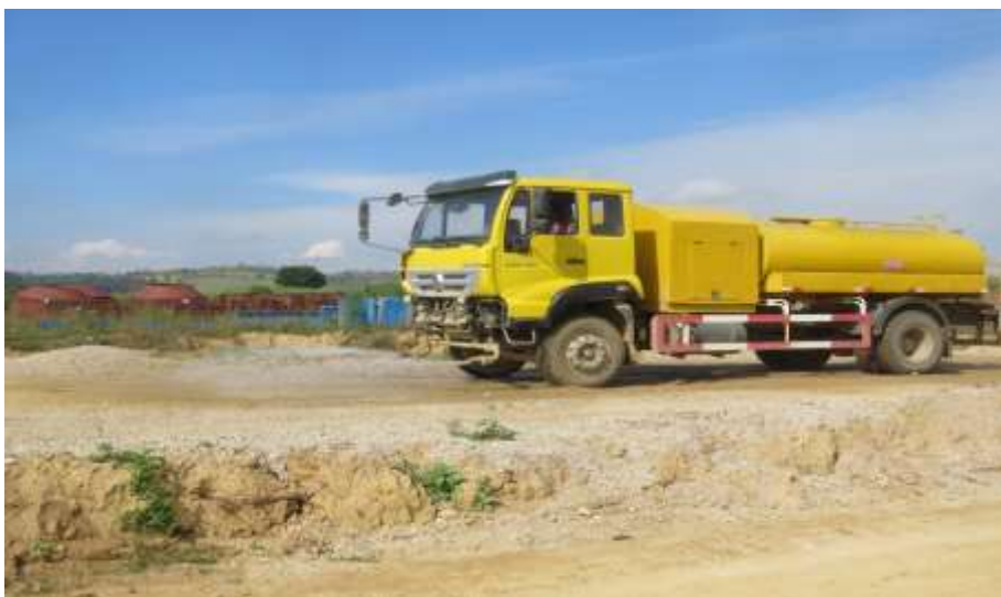
Figure – 26: Spray water for suppression of dust
