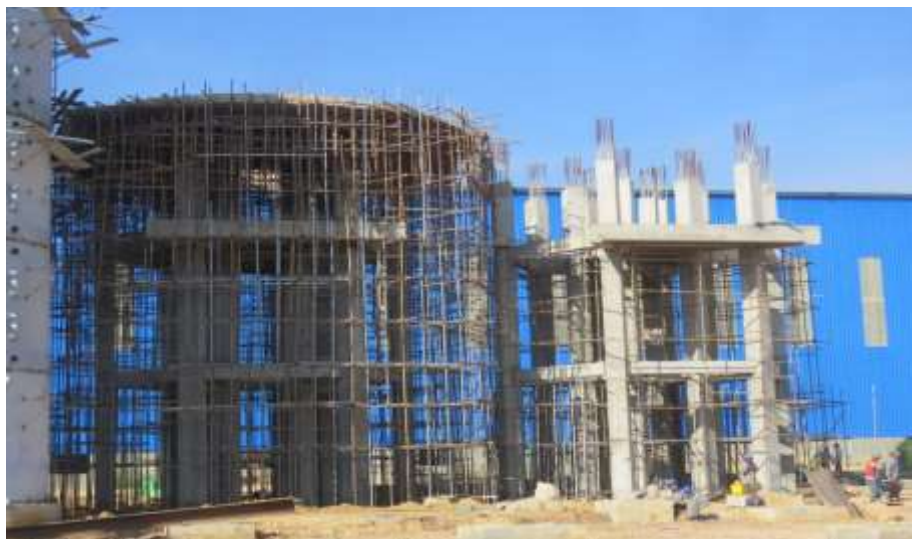
Figure – 16: Clarifier in the process of construction
