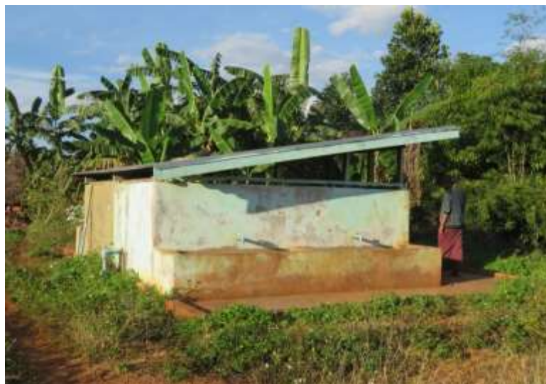
Figure – 58: Community water pond at Palaung Kone village
