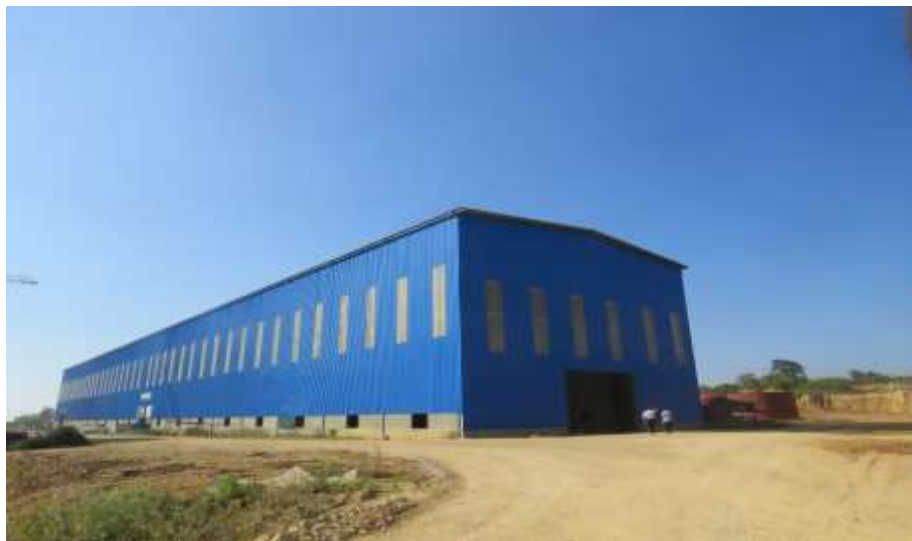
Figure – 12: Mill house
