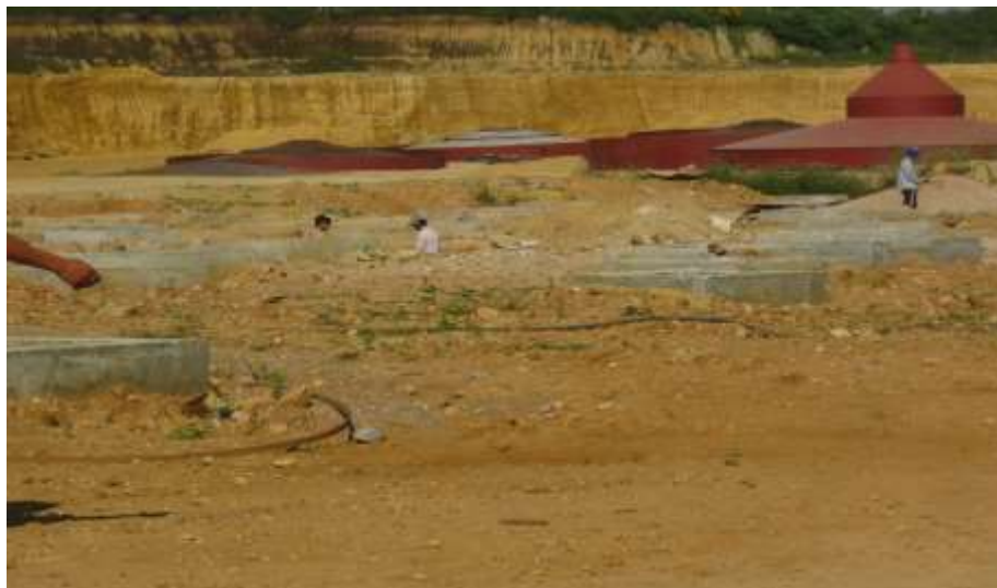
Figure – 15: Evaporation section in the process of construction
