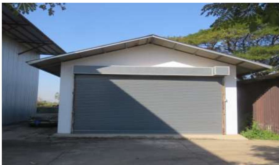
Figure – 24: Light and mirror inspection room
