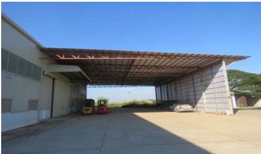
Figure – 26: Loading area
