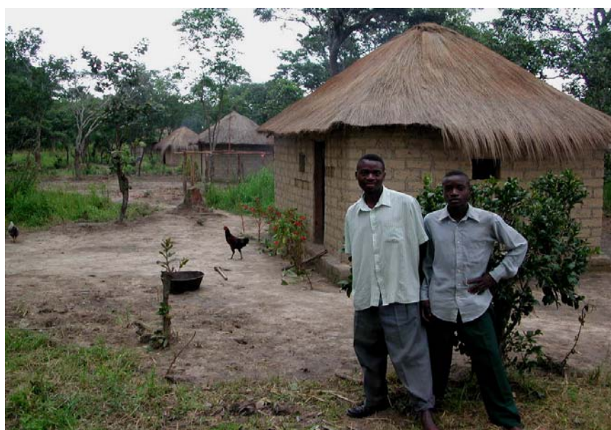
Plate 3.6: Typical adobe brick 'house' or huts construction – Mafuta Village
