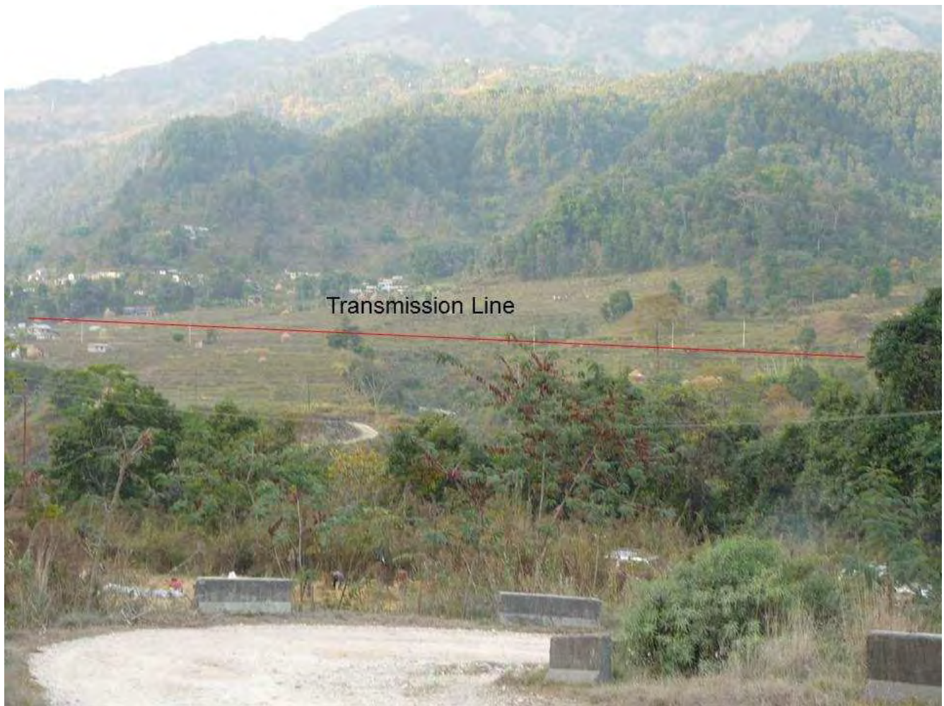
Figure 4: Routing Close to Proposed Udipur Substation Site in Marsyangdi Corridor
