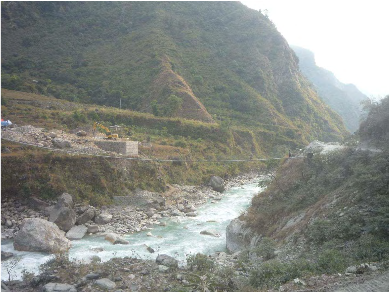
Figure 8: Kaligandaki Corridor - Early Stage Construction Activities for Mistri Khola Hydro. Site is about 2 kilometers north of Tatopani Hot Springs. Land on left side of river is in the ACA (see next photo).
