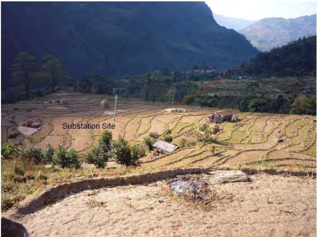
Figure 6: Khudi Substation Site in Marsyangdi Corridor – Site is just inside the ACA
