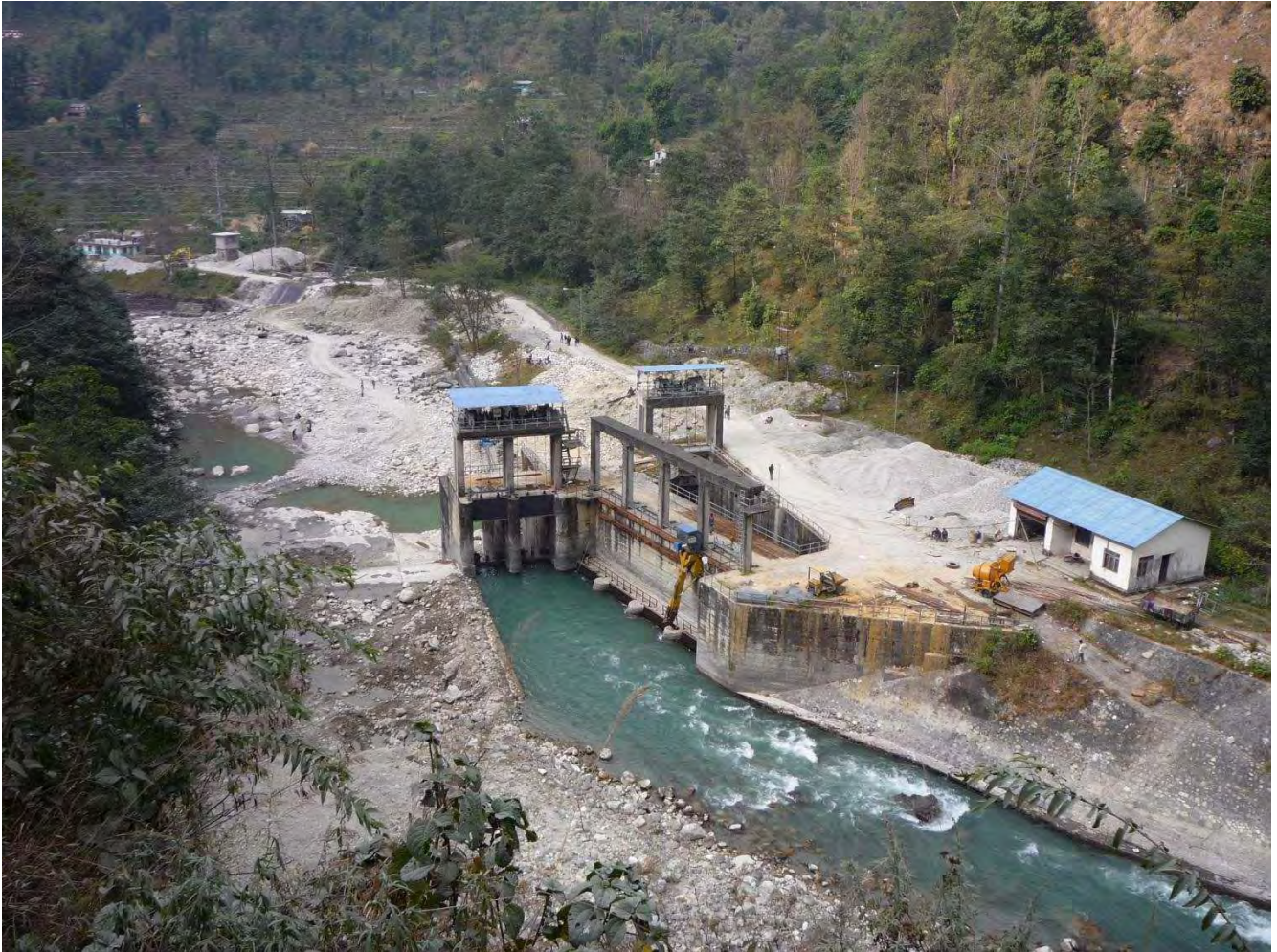
Figure 12: Common Run of River Hydro Plant – Diversion structure of Modi HEP
