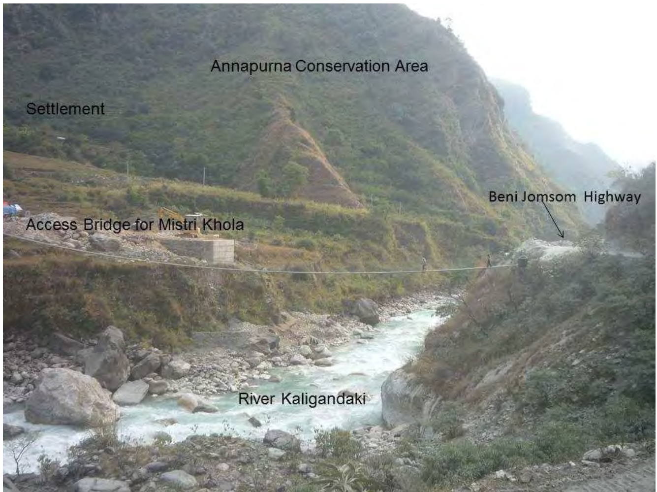
Figure 9: Mistri Khola Hydro Power Construction Kaligandai Corridor
