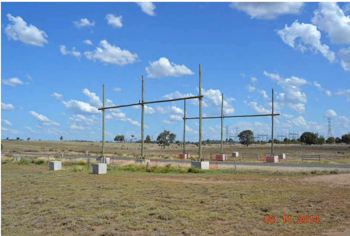
Plate 4: Typical Wood-frame Stringing Hurdle
