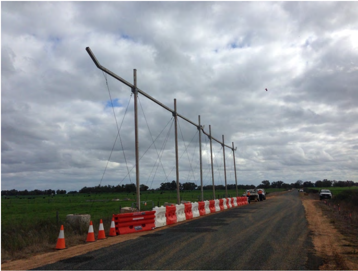
Plate 3: Typical Metal-framed Stringing Hurdle
