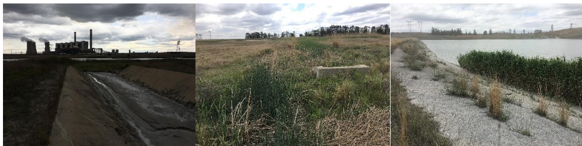
Figure 3: Photographs illustrating stormwater canals entering AD1 and AD2 (left and middle, respectively) and the dam wall at AD3 (right).
