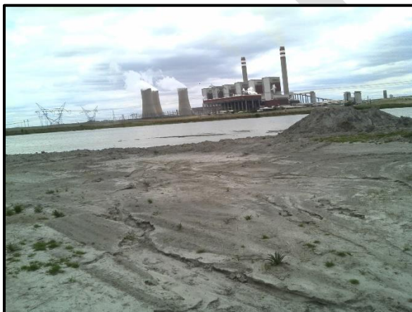
Figure 6. General site conditions
