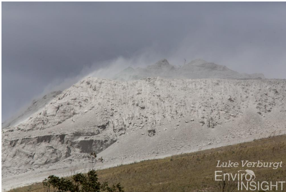
Figure 3-2: Strong winds at Majuba Power Station blowing ash off the ash dump into the surroundings.
