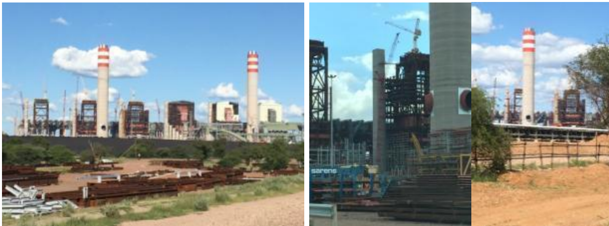
Ongoing construction of the MPS
