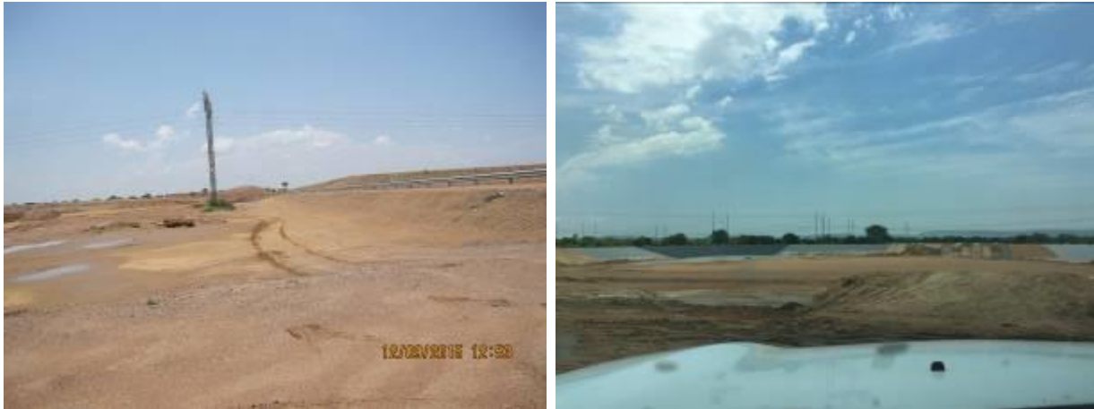
Ongoing construction of the ADF
