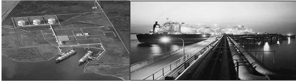
Figure5. Receiving terminal artist's rendering of docks, transfer lines, and storage tanks ( www.cheniere.com )
