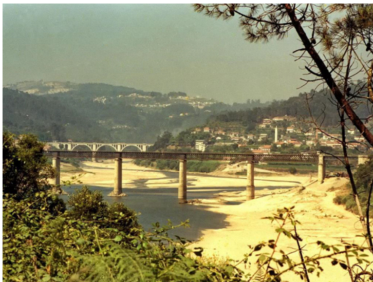
Figure 1. The bridge “Hintze Ribeiro” in Entre-os-Rios, Portugal (1997).
