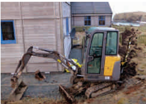
Plate 10. Laying the new electricity cables in the Obs garden, 13th March 2018. © David Parnaby
