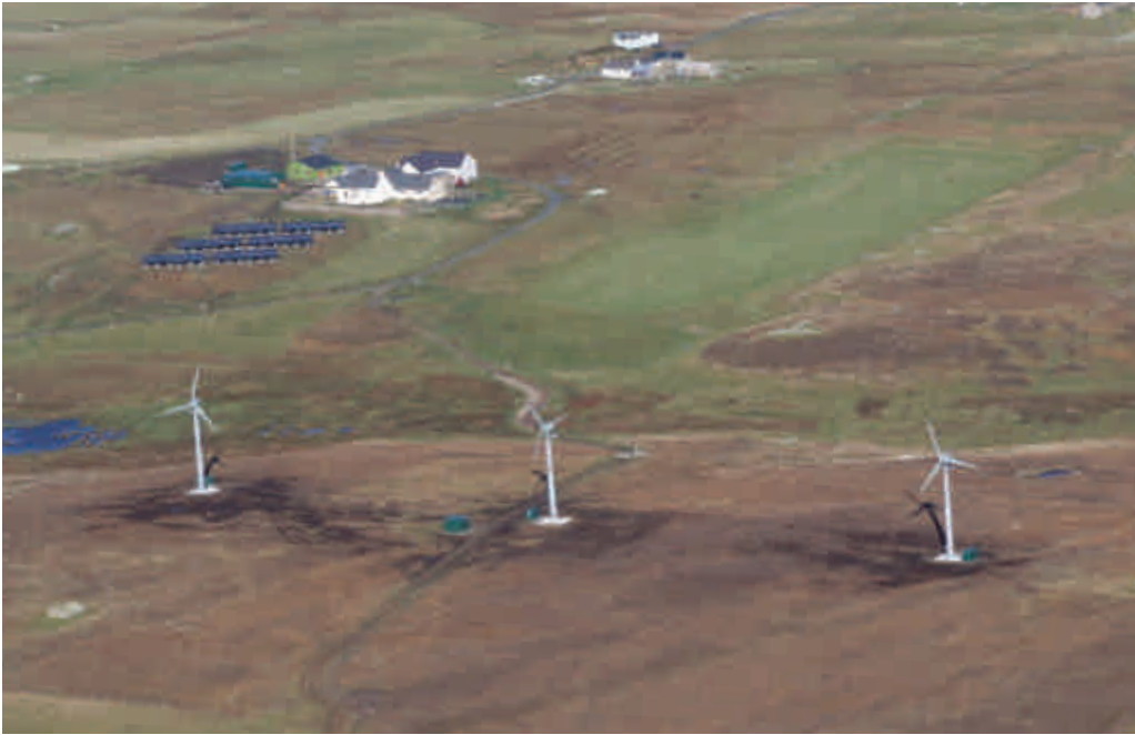
Plate 8. The three new wind turbines on Rippack (left to right, Lukki Minni, Grotti Finni and Tushi) and solar panels on School Brae, 15th October 2018. The dark green building left of the School houses the battery storage and control units. The green shed to the left of Grotti Finni is Tangi. © Ian Andrews
