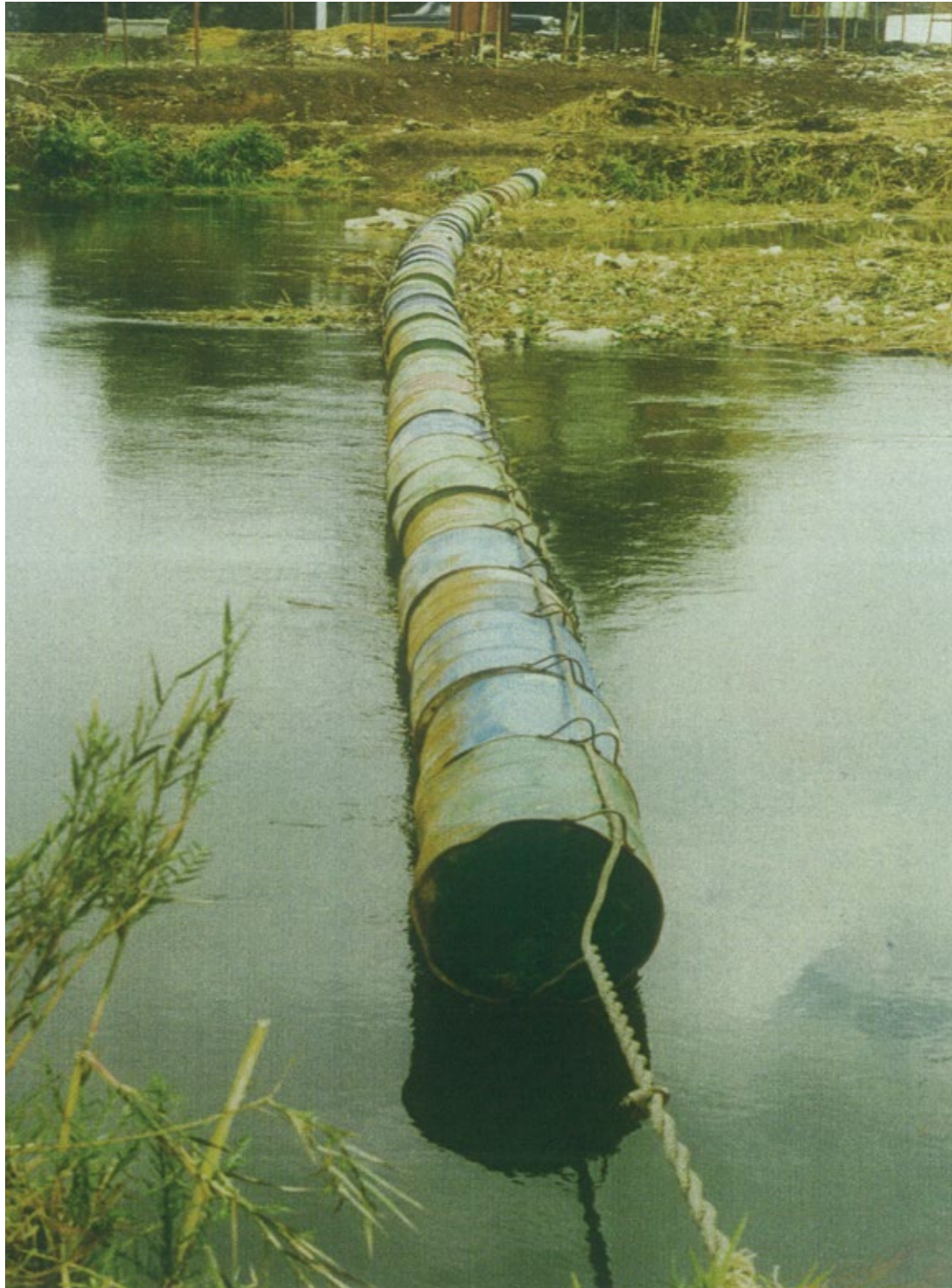
Figure 14. Floating barrier upstream from the Al Mansoureira Canal
