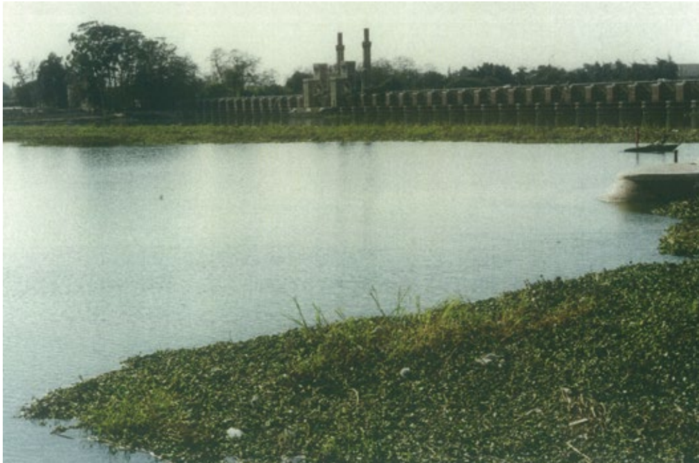
Figure 12. Water hyacinth upstream Damietta Barrage
