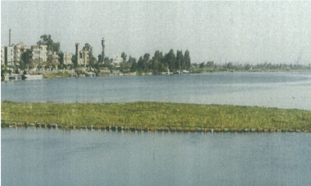
Figure 10. Floating barrier upstream from the Damietta Barrage
