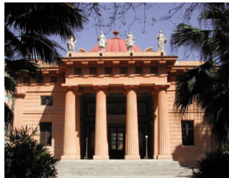
Fig. 3 Main front of the Gymnasium of the Botanical Garden.
