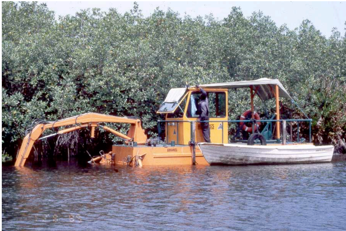
Figure 2. Dredging in mangrove areas of Lower Volta to maintain water access to communities
