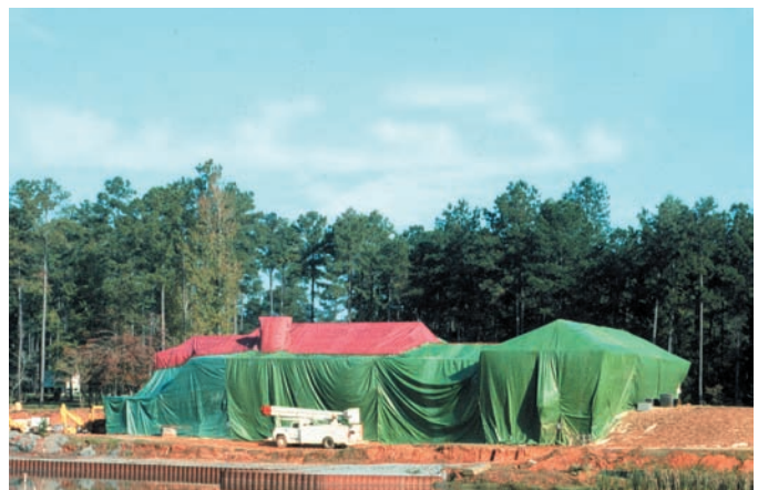
Figure 37 - Fumigating a log home
