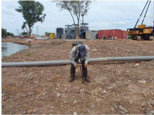
Figure 1. The study site with mixed materials of filled soils
