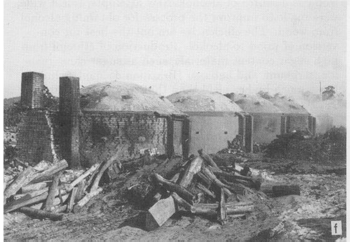
Figure 19-Building of a brick charcoal kiln at La Selva, Veracruz, Mexico (a). Steel charcoal kilns in Venezuela in various stages of operation (b) and assembly (c). Brick charcoal kiln in Venezuela, showing a kiln nearly loaded and ready for bricking shut (d), with door sealed ready for burning (e). Battery of brick charcoal kilns in Venezuela in various stages of operation (f). (M90 0138, M90 0162, M90 0121, M90 0145, M90 0169, M90 0122)
