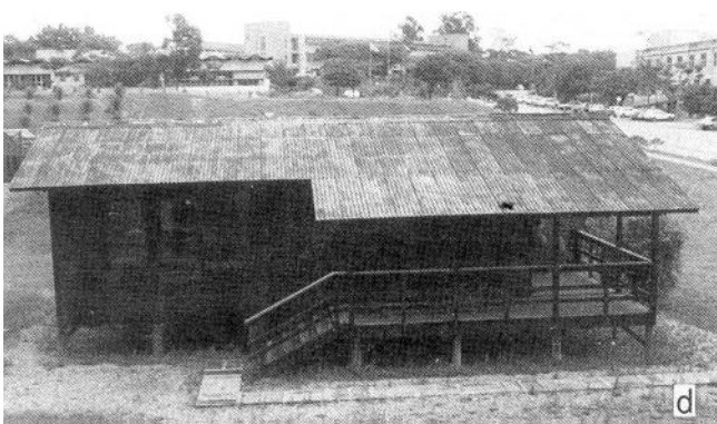
Figure 40-Low-cost house designed by IPT (Instituto Pesquisas de Tecnologicas) Sao Paulo, Brazil. This house is constructed of insect- and decay-resistant Amazonian woods (a). Preservative-treated wood house (b); preservative-treated pine house (c); all native durable wood house (d)—all designed at IPT, Sao Paulo, Brazil. (M90 0156, M90 0109, M90 0133, M90 0157)
