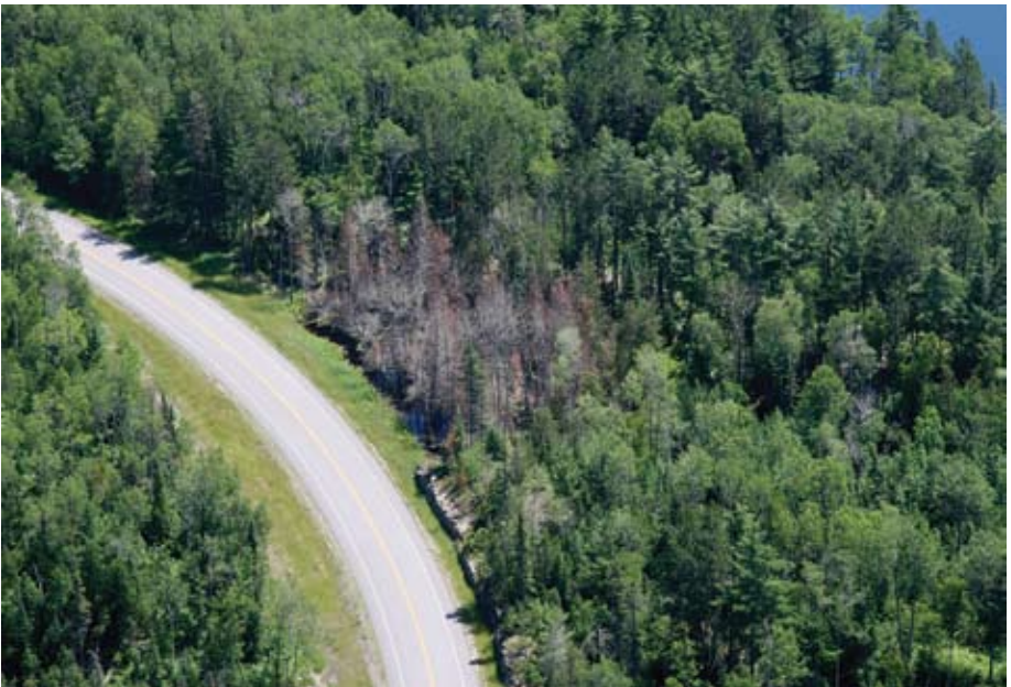
Figure 87. Tree mortality due to inundation caused by a plugged culvert. North of Ely, Superior National Forest, MN.
