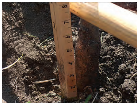
Figure 1-7 —A tree that was planted too deep. The slight bulge at the base of this budded tree should have been above the soil surface (John Ball South Dakota State University, used with permission).
