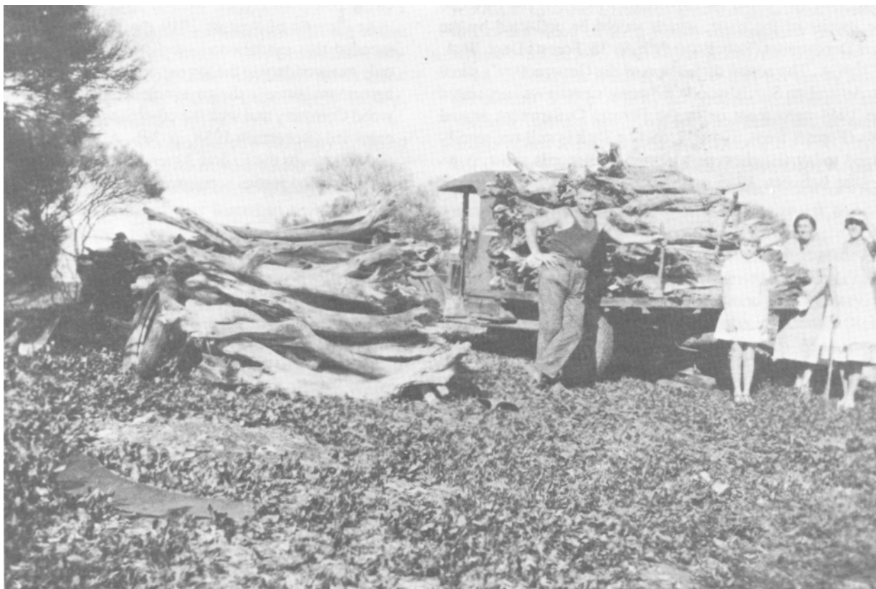
Figure 3 —After the war, transport of larger logs over greater distances was made possible by motor vehicles. Photo: Neil Mitchell, Battye Library, Western Australia.
