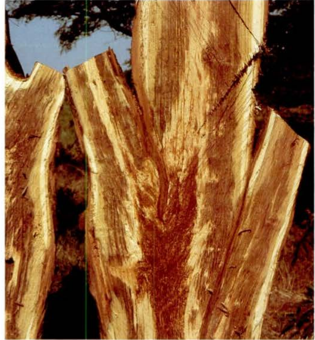
Figure 38-5. Longitudinal section of black locust with wood decayed by P. robineae .
