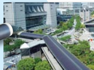
Film-Type Solar Cells Film-type solar cells are "lightweight, thin and flexible," and are installed in the arched roofs over the moving walkways in Minato Mirai 21 district in Yokohama, Kanagawa Prefecture, and are able to supply roughly 20% of the annual electricity used by the walkways.
