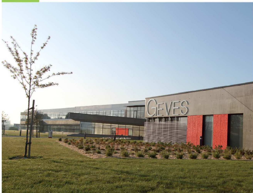
The GEVES site in Beaucauzé combines the head office, the National Seed Testing Station, and part of the BioGEVES laboratory.
