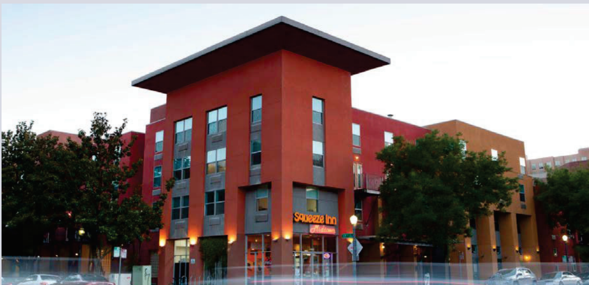
Pensione K Affordable Apartment Complex
