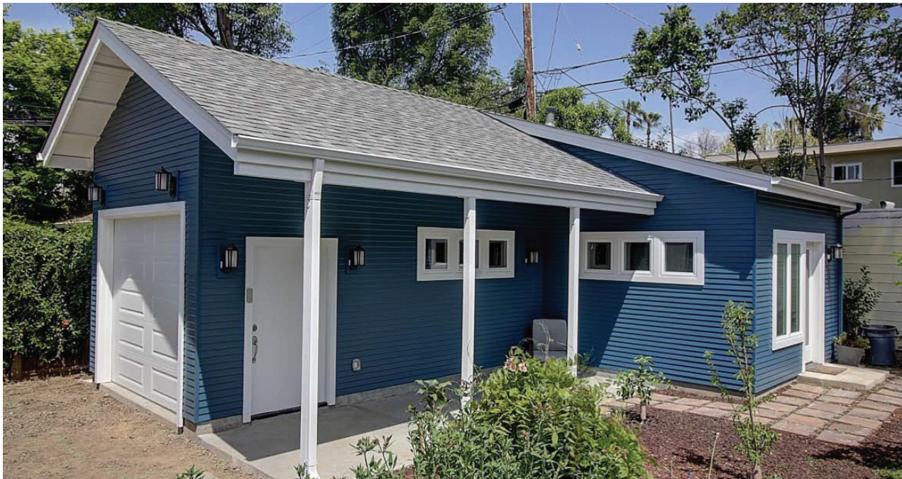
Example of an Accessory Dwelling Unit Attached to a Remodeled Garage
