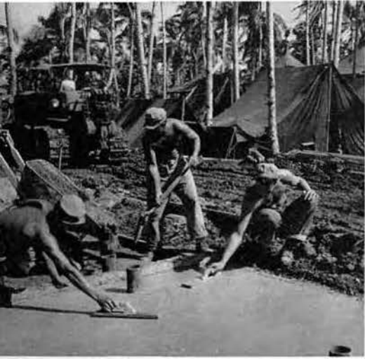
Concrete crew laying deck
