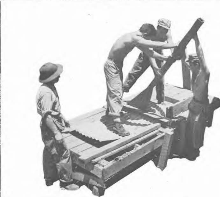
Our own invention for cutting Quonset Hut sheet metal
