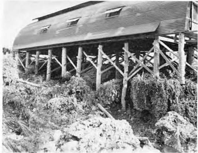
The terrain was a great obstacle to construction
