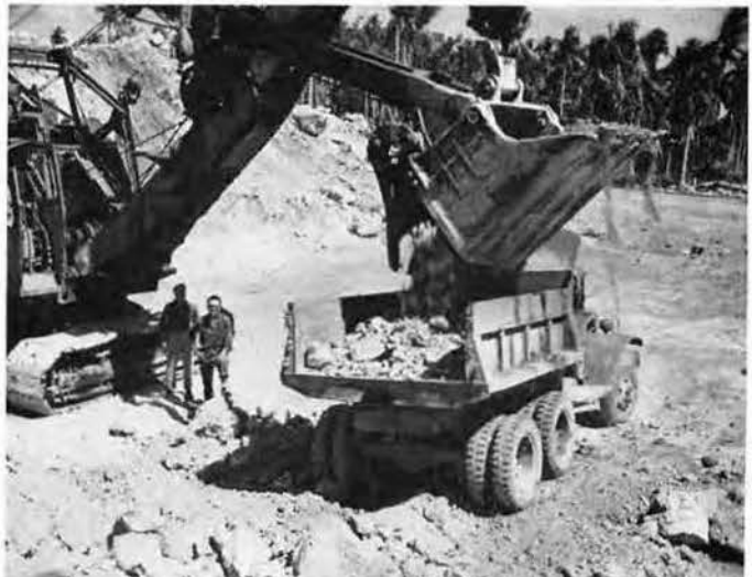
The coral pits were busy day and night
