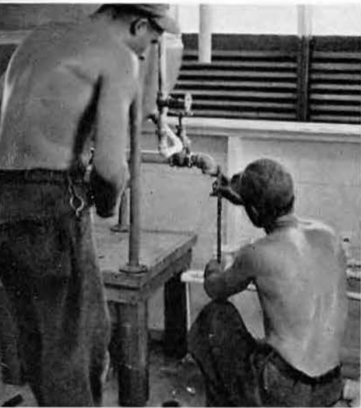
Modern installations by our plumbers—Naval Base Galley
