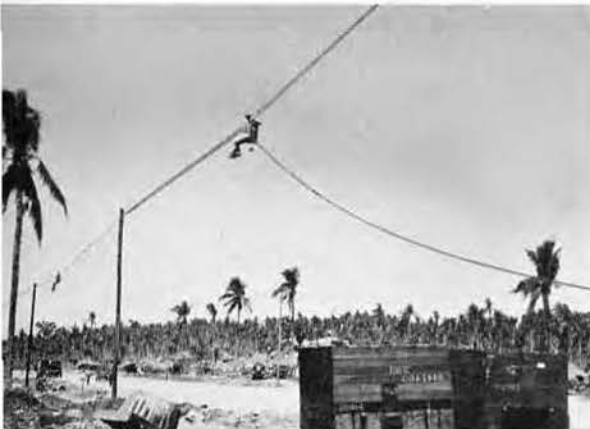
Telephone linemen at work
