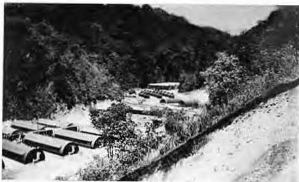
A portion of the Hollandia Hospital
