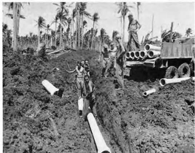
The pipe crews laid miles of water main
