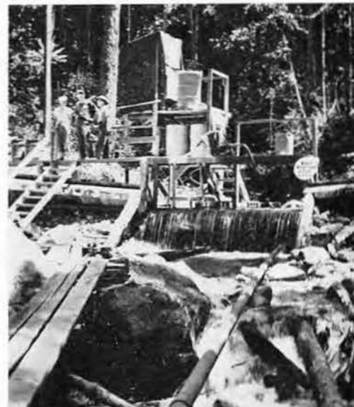
Dam for hospital water supply
