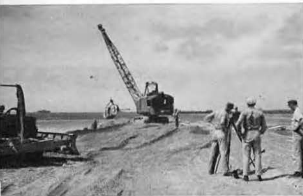
Depickling Jetty Construction
