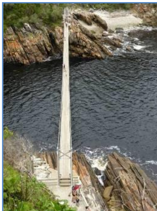
Storms River suspension bridge.
