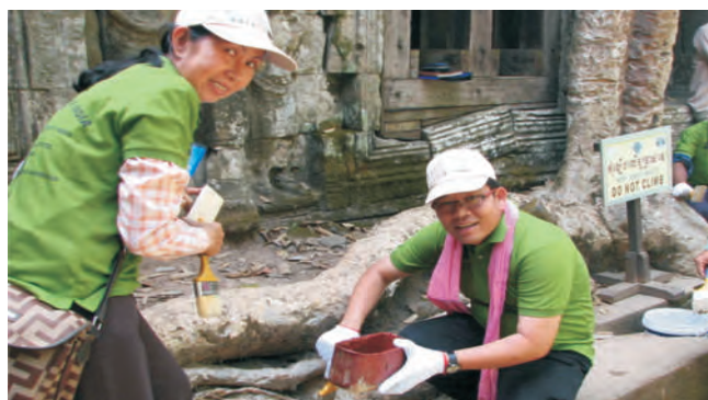
Treatment of Trees at Ta Prohm Temple, Cambodia
