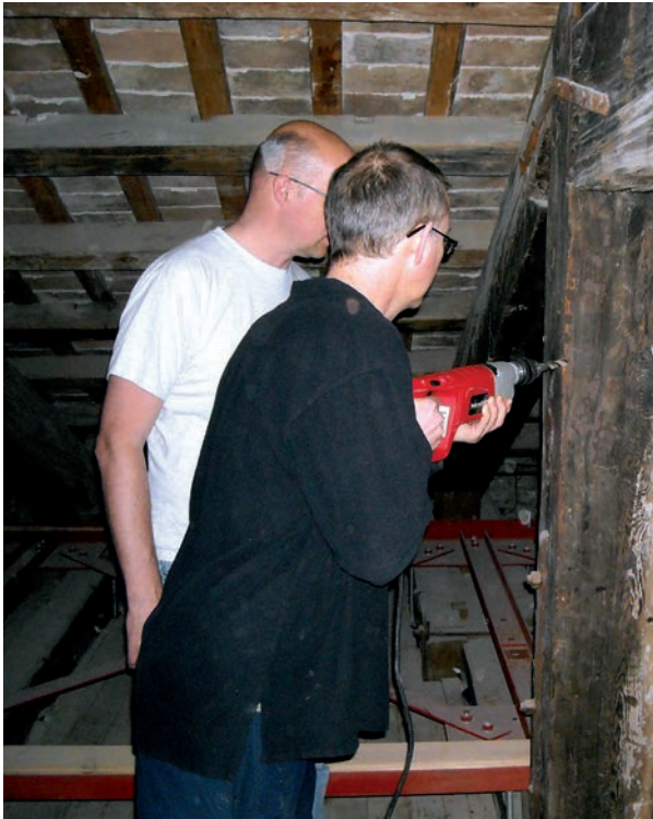
Photo 3/ Coring historic timbers with a drill-mounted borer.
