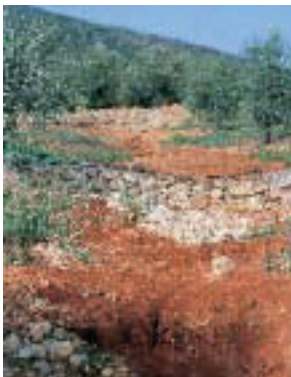
Figure 32. Gabions packed with stones designed to slow down water velocity.
