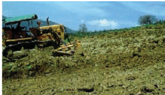
Figure 20. Levelling the site.
