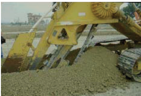
Figure 23. Digging and laying drainage pipes.
