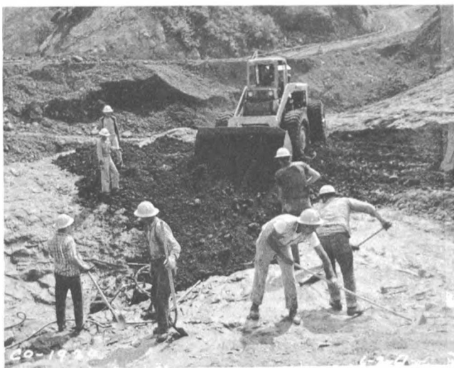
(B) ...and then initial lift of core material is placed
