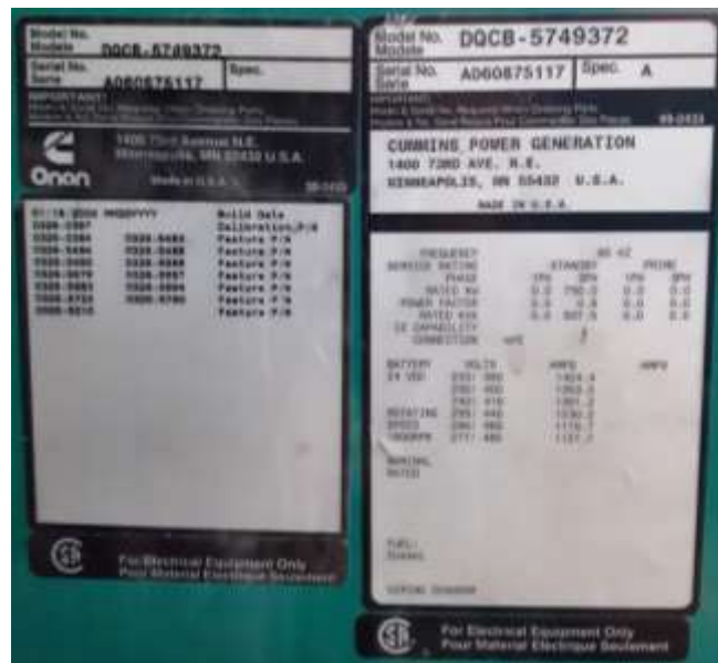
Figure 2: Example of Generator Name Plates
