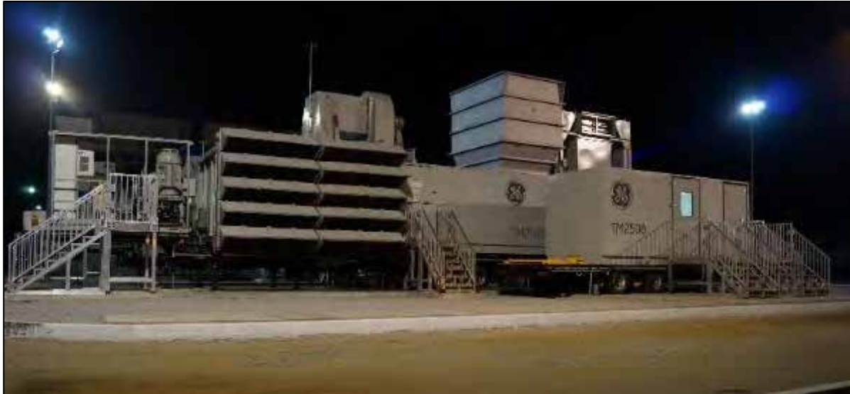
Photo 5-25: Xitoto thermal power plant with the operation of the TM 25000 GEN turbine.
