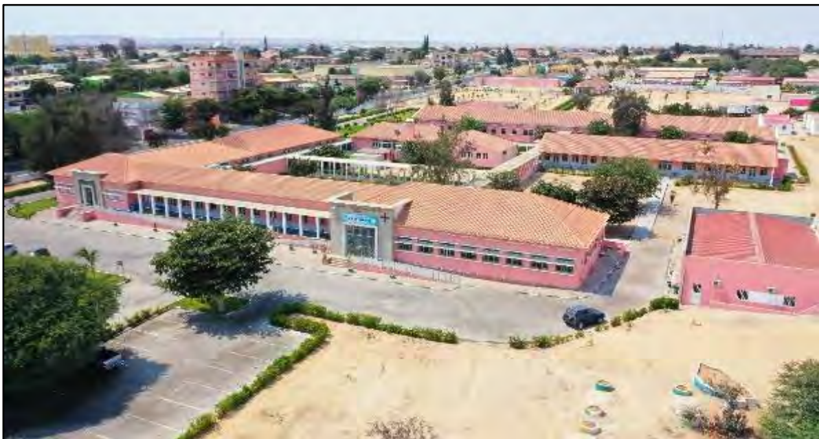
Photo 5-27: Provincial Hospital of Ngola Kimbanda in Moçâmedes.
