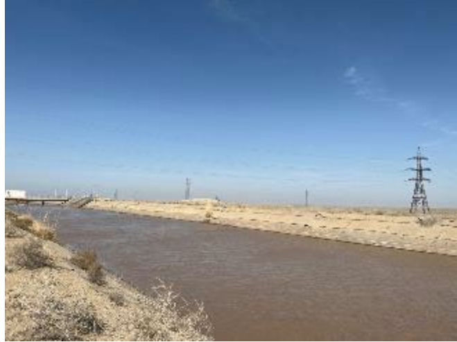
Figure 41: Existing OHTL crossing the irrigation channel
