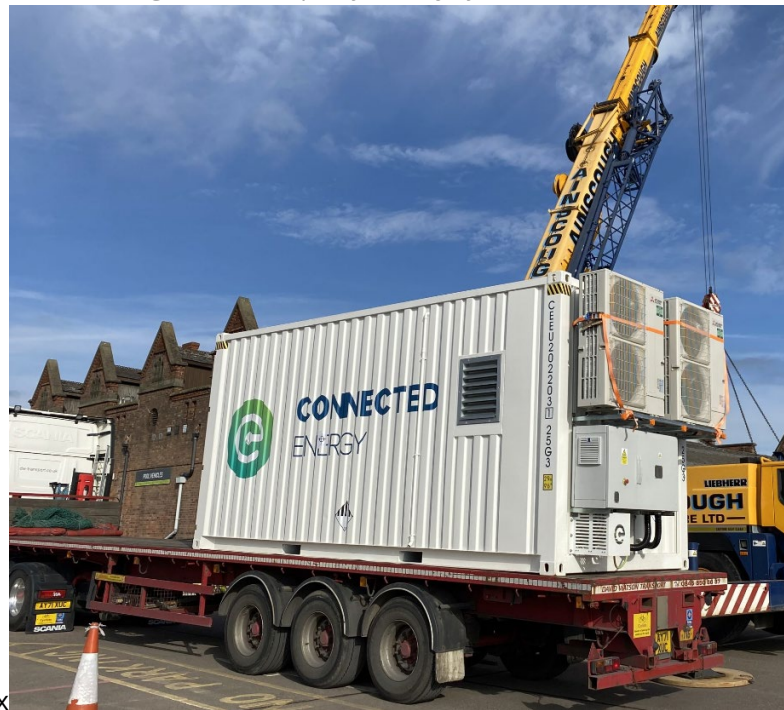
Figure 94: Example of delivery of BESS containers
