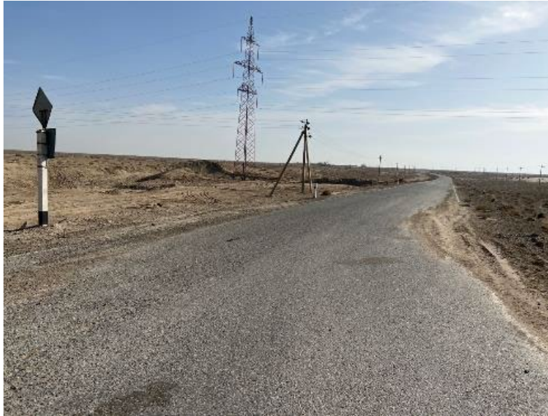
Figure 28: Existing R78 (photo)
