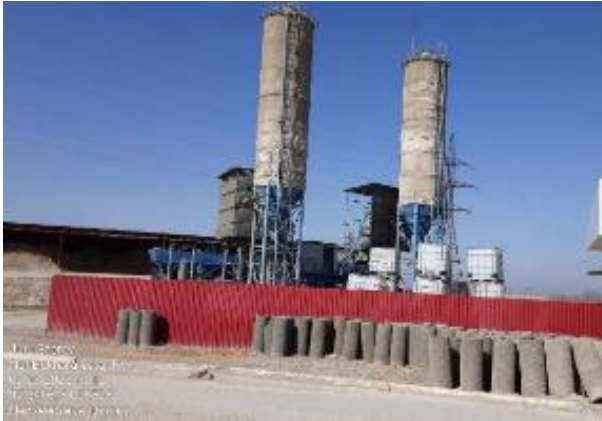
Figure 44: Photo of the batching plant
