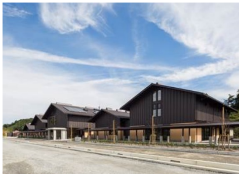
Nobiru civic center newly opened on a hill after relocation (Materials of Higashimatsushima City)
