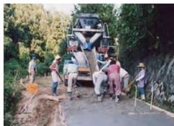
Road improvement by residents of Shimojo-mura
