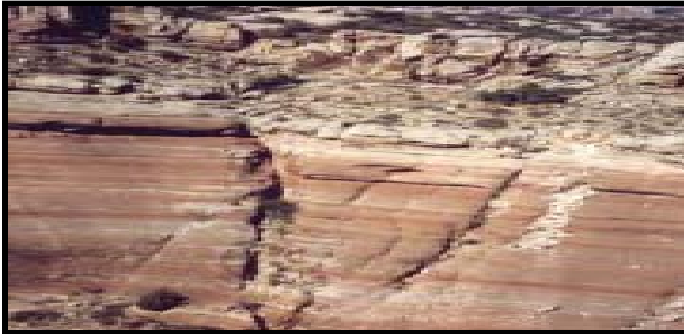
Figure 4: Studied fault system at location 1; Road cut along the Expressway to Onitsha
