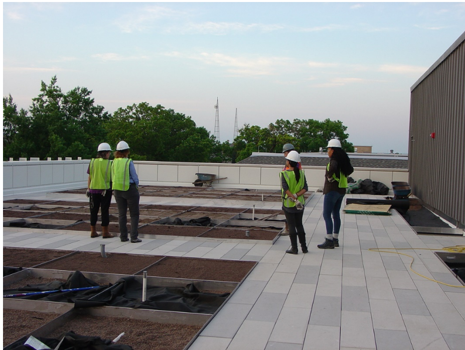
APDesign Experimental Green Roof Beds being installed by contractors working with green roof installers from Blueville Nursery. Summer of 2017
