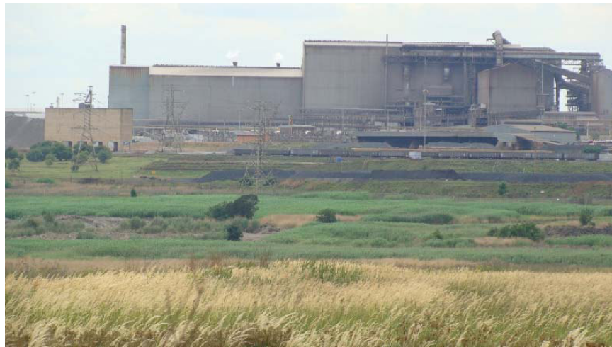
Figure 2: View across Vaalbank Spruit wetland towards Samancor industrial complex with the southern tip of slag dump amongst reed beds on the left.
