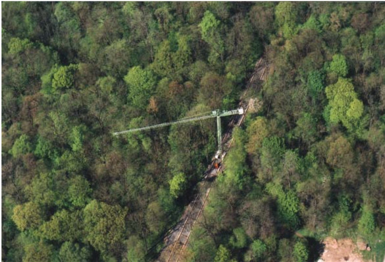
Figure 3.2: The Leipzig Canopy Crane in spring (source: LAK project)
