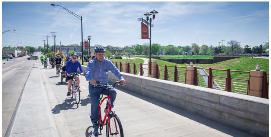
Cycle Track Integrated into Vehicular Bridge
