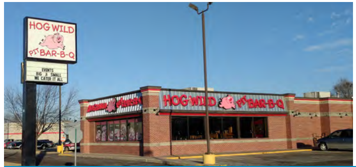
Single Tenant, Single Story Building
