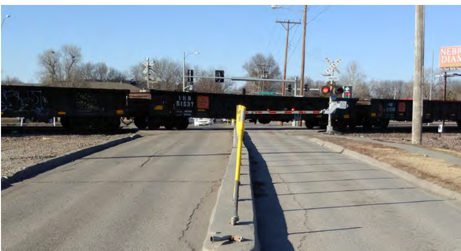
Intersection of North 44th Street and BNSF Railroad
