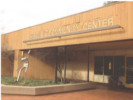
② Community Center main entrance
