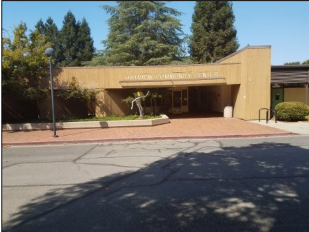
Exterior of the existing Hillview Community Center.
