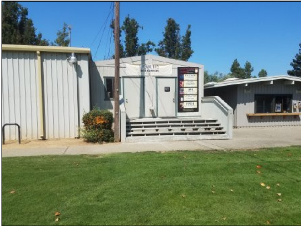
Exterior of the Bus Barn Theater building with ticket office and other outbuilding.
