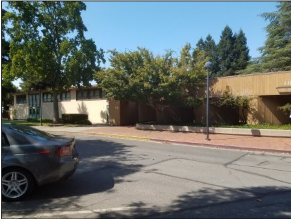
Exterior of the existing Hillview Community Center.
