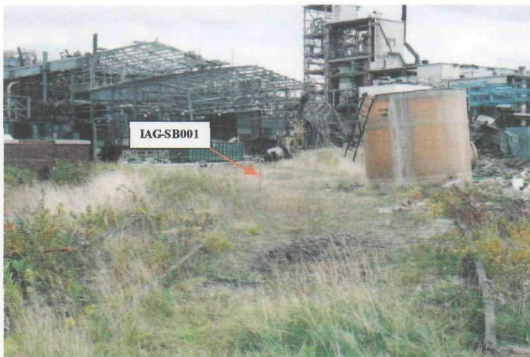
Photo # 37 (Sept. 21, 2000; time: 1605; Roll 2, Sequence 22) Boring Location: IAG-SB001 ; West of Bld. 428 in Area G: Facing SE
