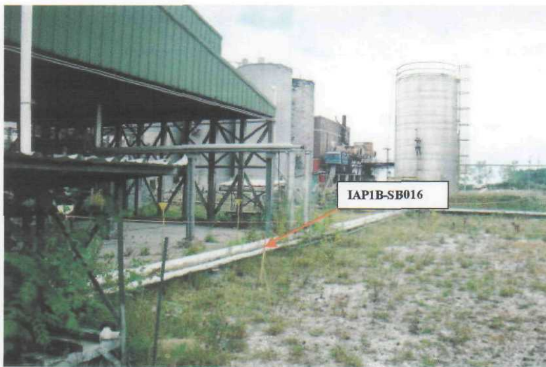
Photo # 16 (Sept. 21, 2000; time: 1455; Roll 1, Sequence 19) Boring Location: IAP1B-SB016 ; East Side of MDI/TDI Transfer Sta.; Facing north
