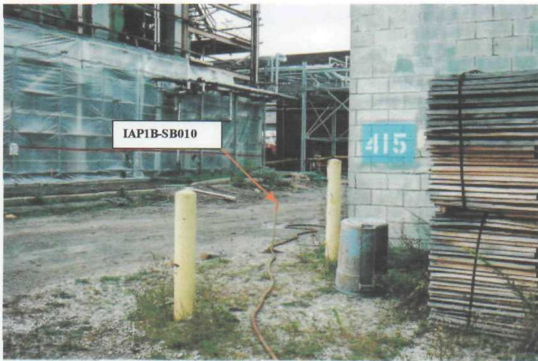
Photo # 10 (Sept. 21, 2000; time: 1456; Roll 1, Sequence 20) Boring Location: IAP1B-SB010 ; West of Bld. 415; Facing NW
