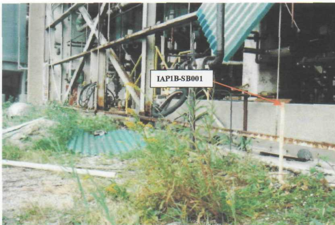
Photo # 1 (Sept. 21, 2000; time: 1440; Roll 1, Sequence 11) Boring Location: IAP1B-SB001 ; West Side of Bld. 414; Facing NW
