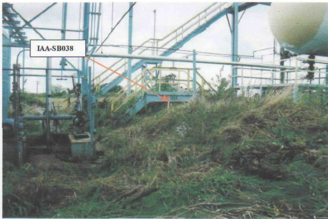
Photo # 29 (Sept. 21, 2000; time: 1532; Roll 2, Sequence 14) Boring Location: IAA-SB038 ; South of BDE Tank in Area A: Facing NW
