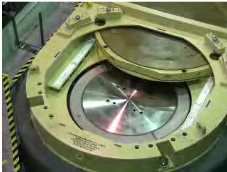
Figure C-13: Canister Lowered into Overpack; Lift Cleats and Downloader Slings Removed
