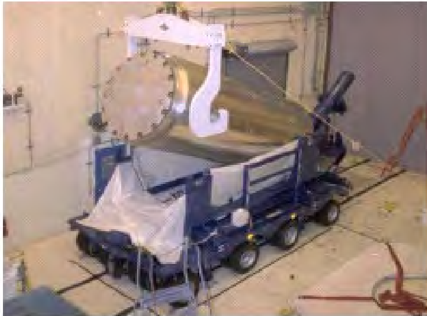
Figure C-3: Lowering Cask onto Trailer
