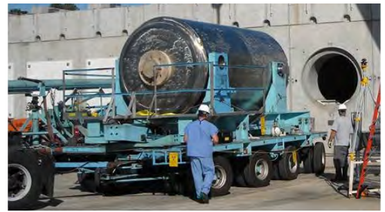
Workers prepare to load an AREVA-TN NUHOMS canister into a concrete storage module at the Calvert Cliffs Nuclear Power Plant in Lusby, MD. (Courtesy: Exelon)
