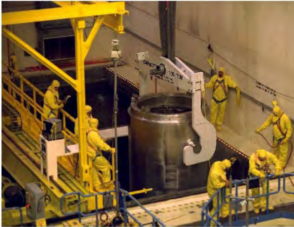
Figure 6. Canister and Transfer Cask Being Decontaminated
