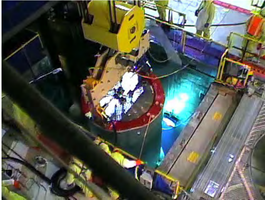
Figure C-6: Transfer Cask and Canister Lowered into Spent Fuel Pool
