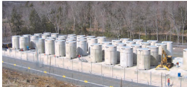
Loaded spent fuel storage casks are in place on storage pad at the Haddam Neck Plant in Meriden, CT. (Courtesy: Connecticut Yankee)
