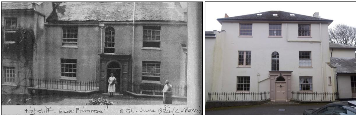
(l) Rear Elevation with Gulielma Lister (figure on the right) in 1924 (from her Thesaurus) and (r) in 2013, with the upper storey added in 1936.
