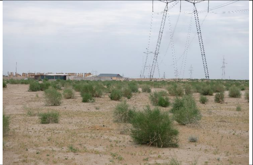
VP 15. Degraded area near the Karakul substation. Residential buildings, roads, pit, garbage, noise. Heavy traffic.
